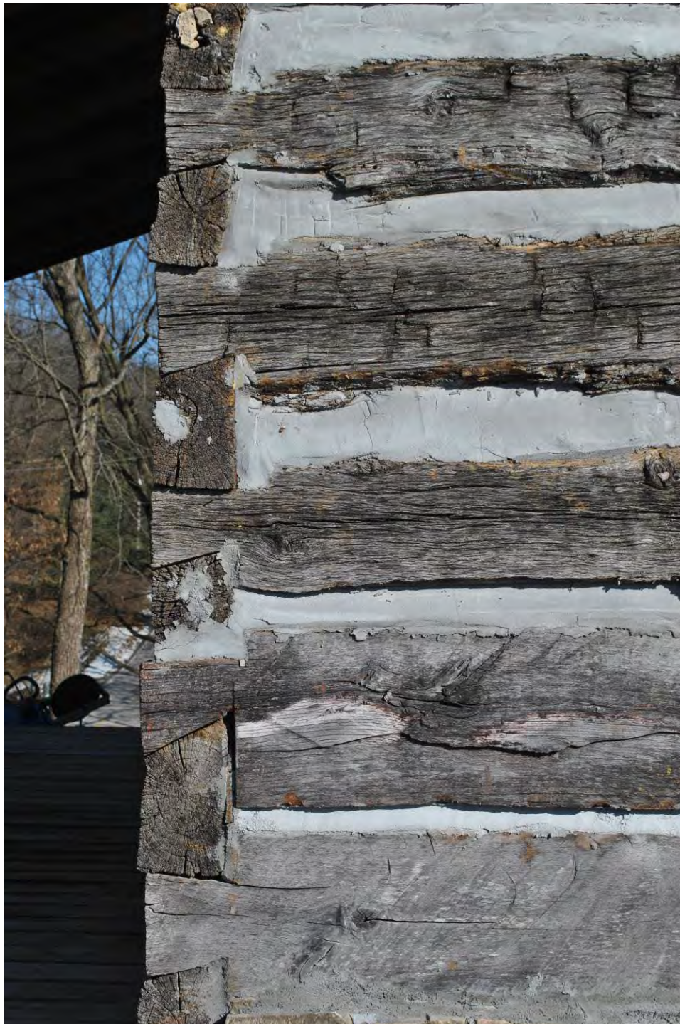
Figure 5: Detail of a series of typical half dovetail notches at the southwest corner of the Roberts Log Cabin (Mason Martel, Rosin Preservation, LLC, February 2024).
