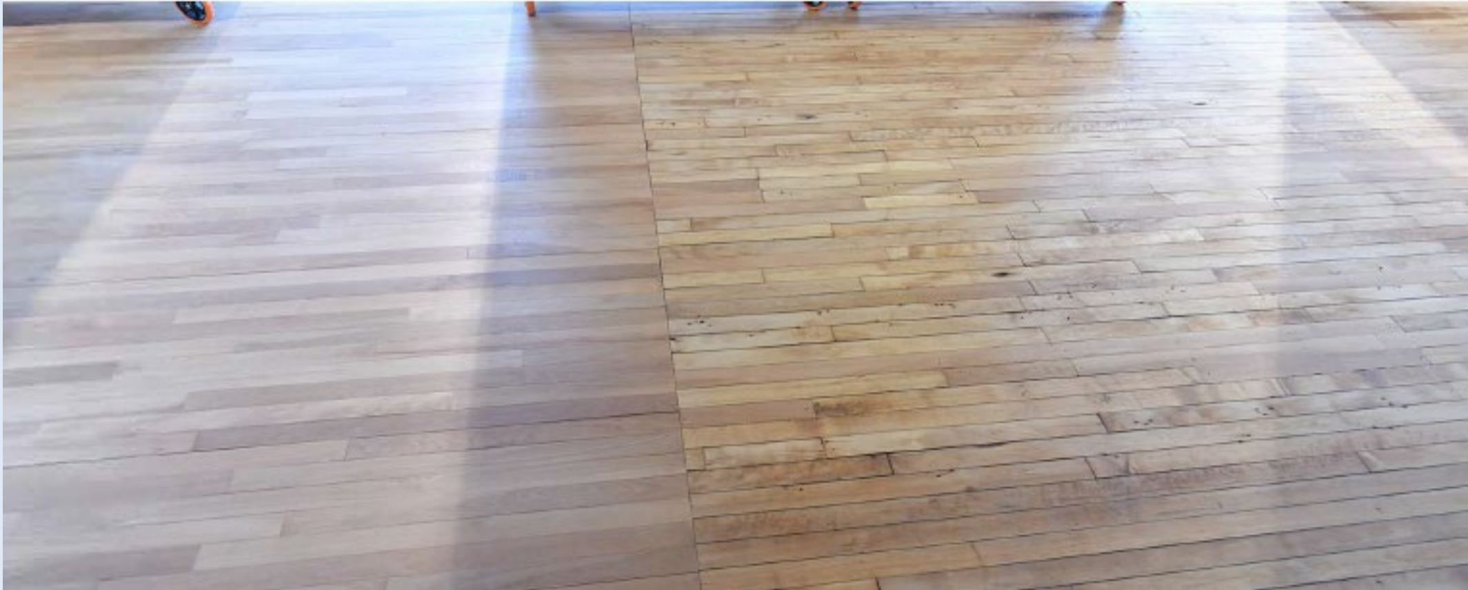
New wood patched in to replace missing wood
