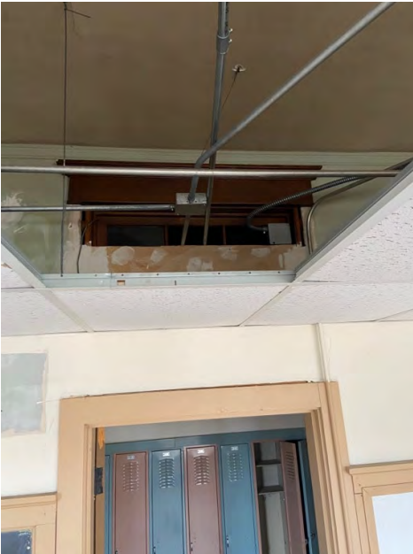
Figure 18: Original transom window visible above dropped acoustical tile ceiling.
