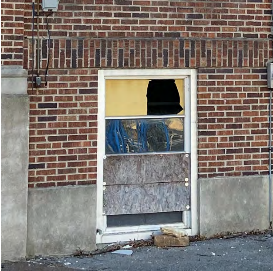
Figure 20: Broken glazing panel on the north elevation of the 1923 building.
