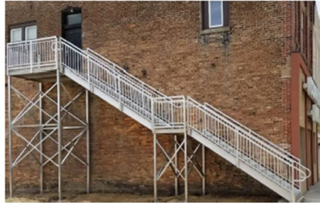
Example of an appropriate fire escape installation. (Upside Innovations)
