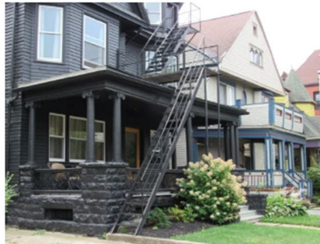
Example of an inappropriate fire escape installation. (The 59 Club Blog)
