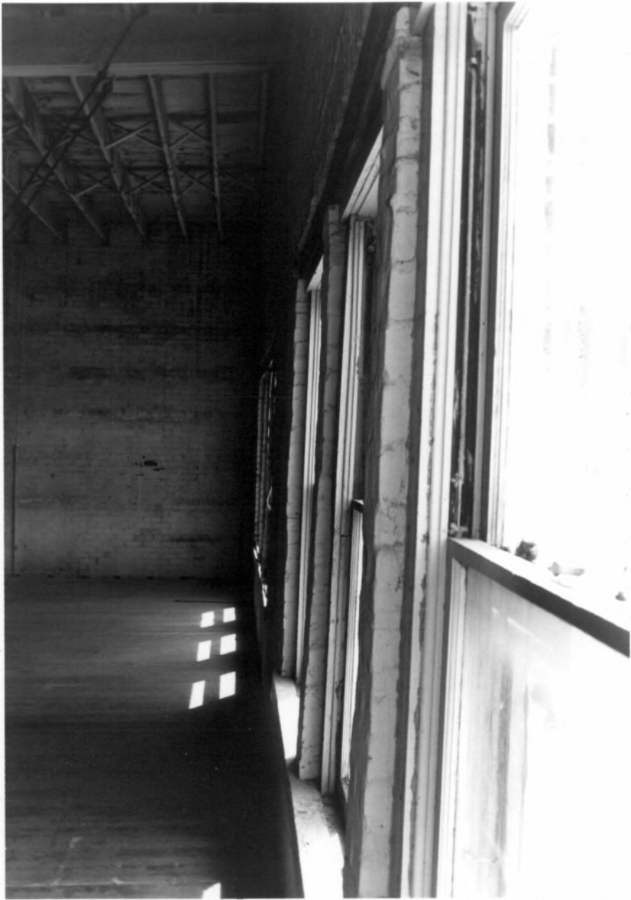
Wire Reed Store Building 438-440 So. Campbell Ave. Springfield, Greene Co., MO Photo 14
