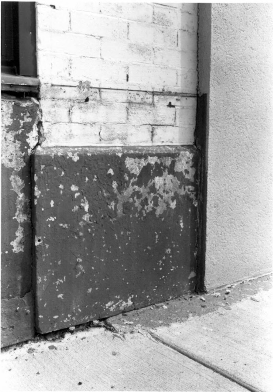
Wise Feed Co. Building Springfield, Greene Co., MO Photo 7
