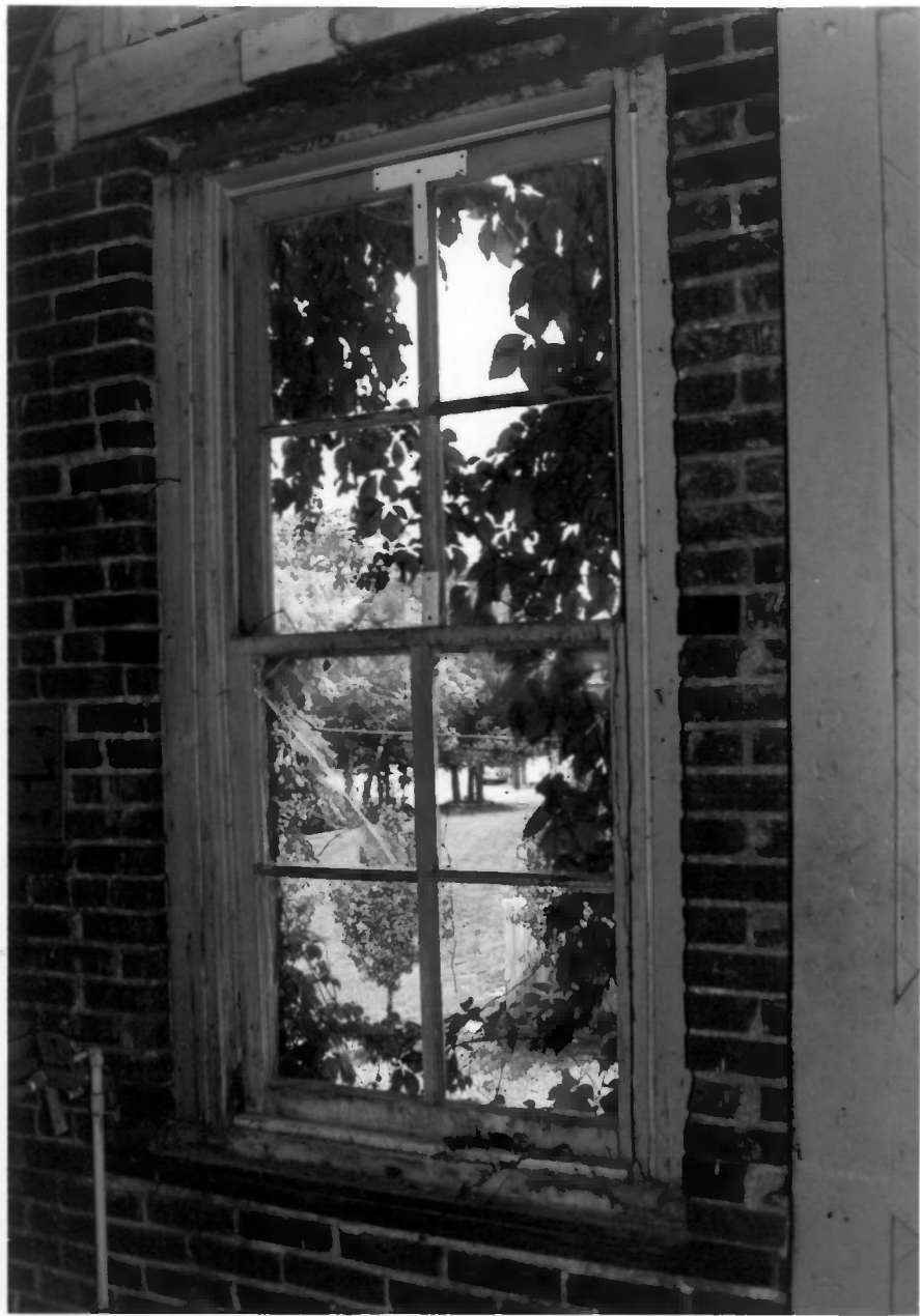
W. & R. Co. Building Springfield, Greene Co., MO Photo 30
