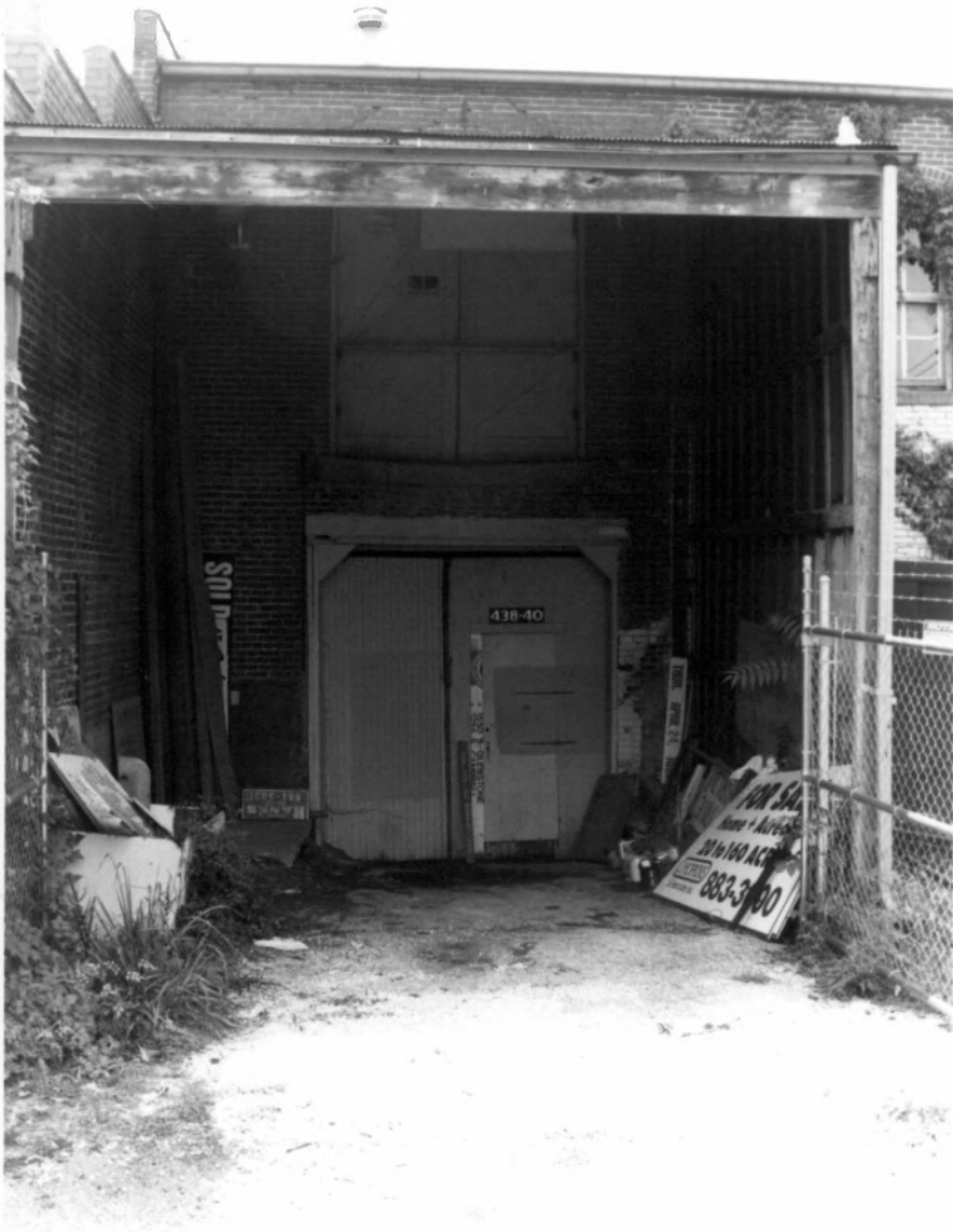
Wise Feed Co. Building Springfield, Greene Co., MO Photo 10
