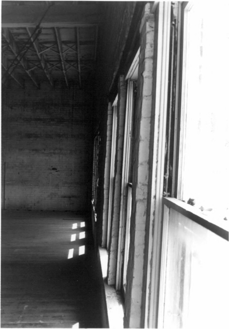
W. H. Reed Co. Bldg. near Springfield, Greene Co., MO Photo 26
