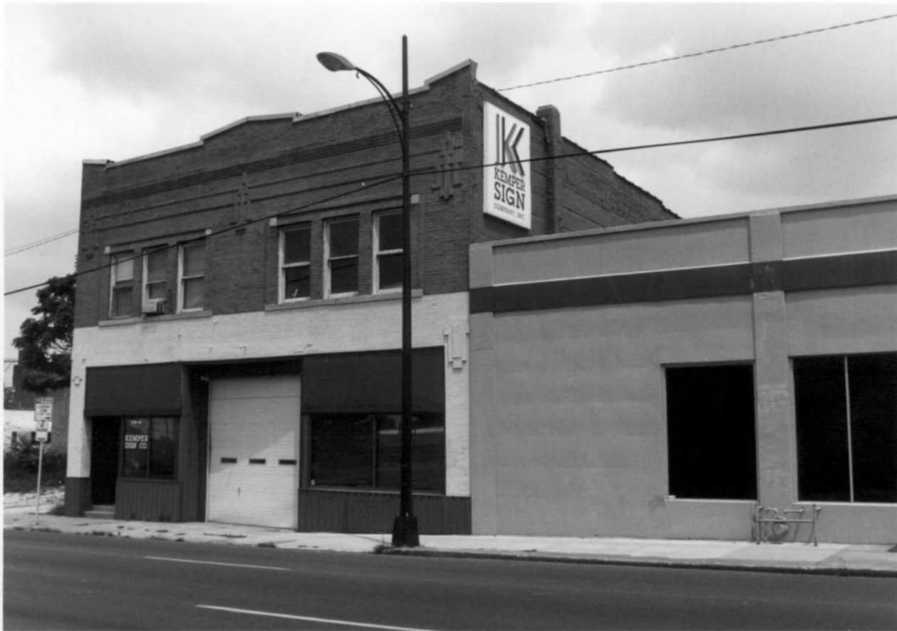
Wise Feed Store Building 438-440 So. Campbell Ave. Springfield, Greene Co., MO Photo 4
