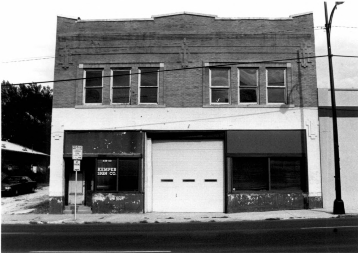
Wise Feed Store Building 438-440 So. Campbell Avenue Springfield, Greene Co., MO Photo 9
