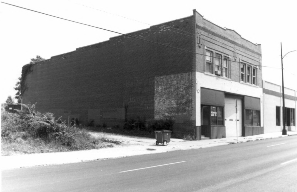
Wise Reed Co. Building
