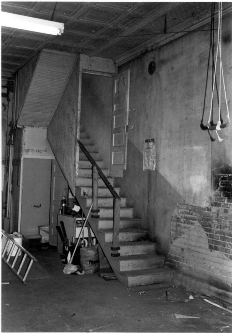
Wise Reed Co. Building Springfield, Greene Co., MO Photo 22
