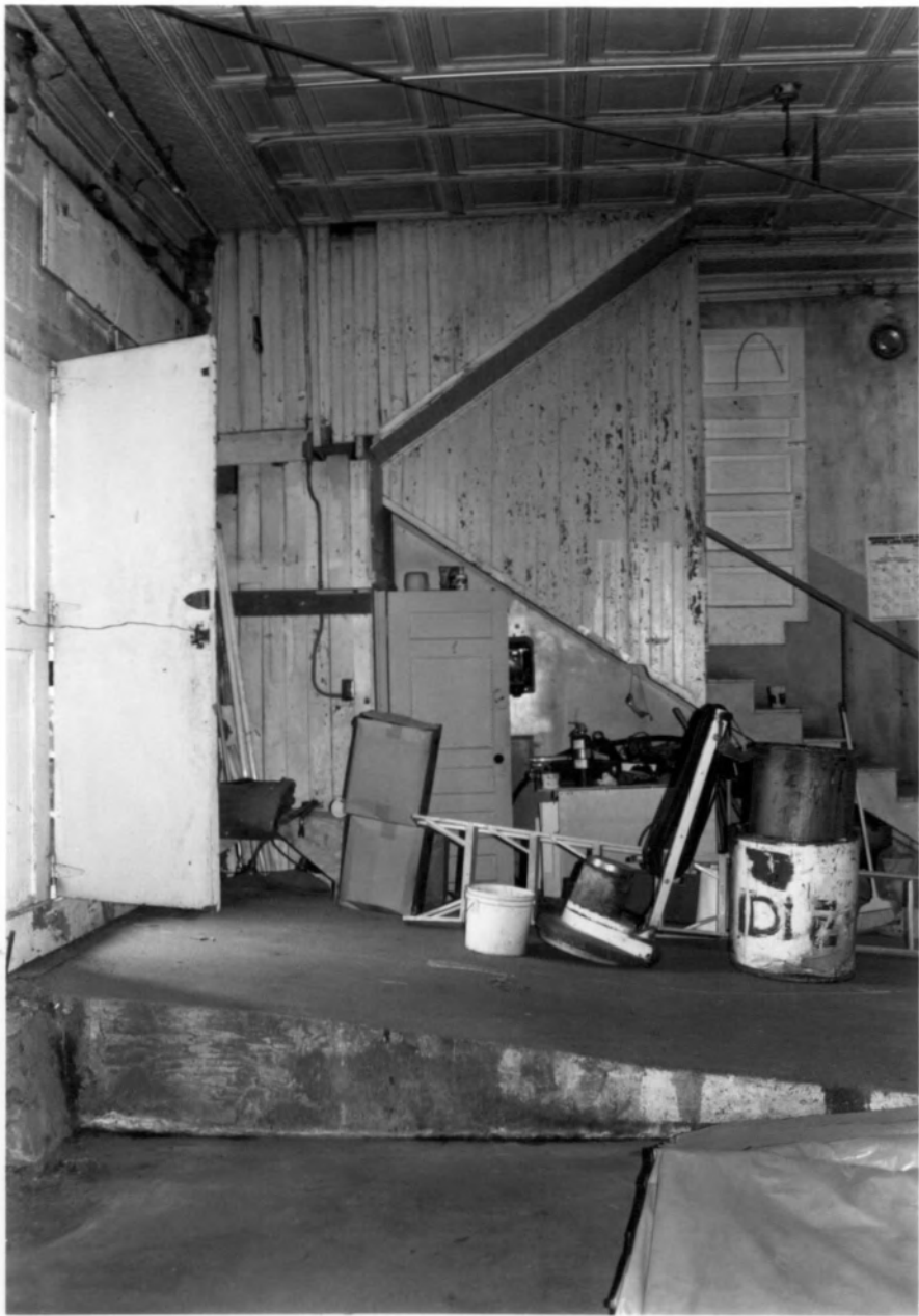
Wire Reel Co. Building Springfield, Greene Co., MO Photo 23
