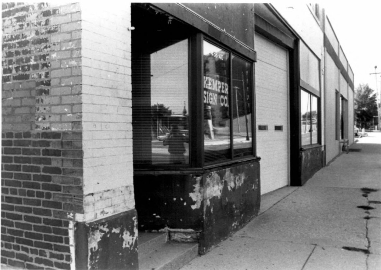
Wise Feed Store Building 438-440 So. Campbell Ave. Springfield, Greene Co., MO Photo 10
