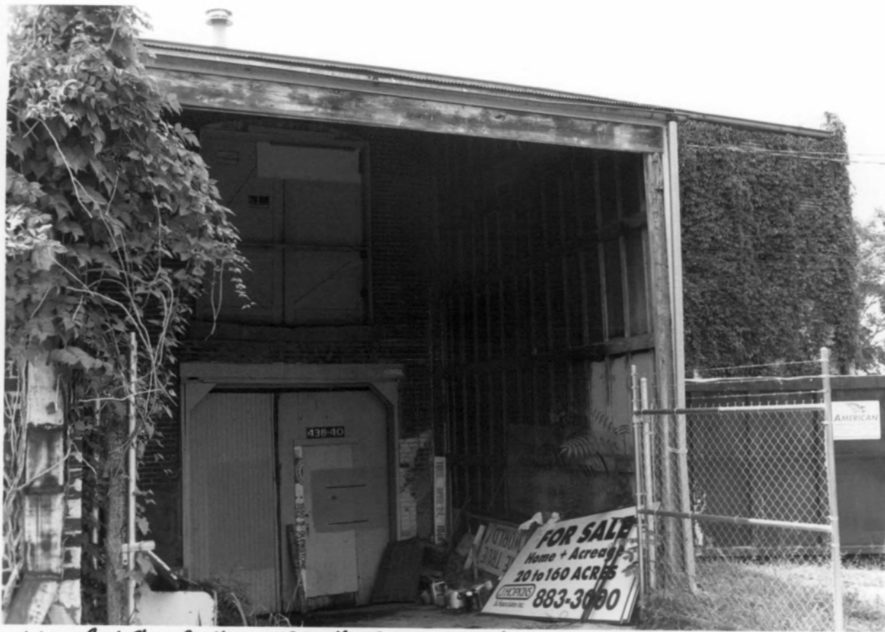
Wise Feed Store Building 438-440 So. Campbell Ave. Springfield, Greene Co., MO Photo 5
