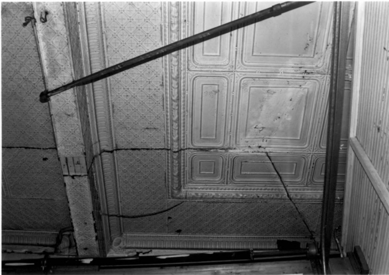
Wise Feed Co. Building
