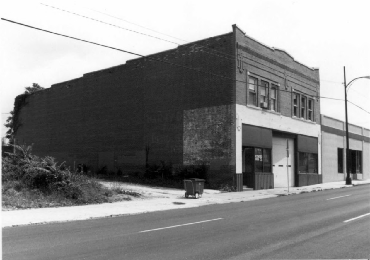
Wise Feed Store Building 438-440 So. Campbell Springfield, Greene Co., MO Photo 8
