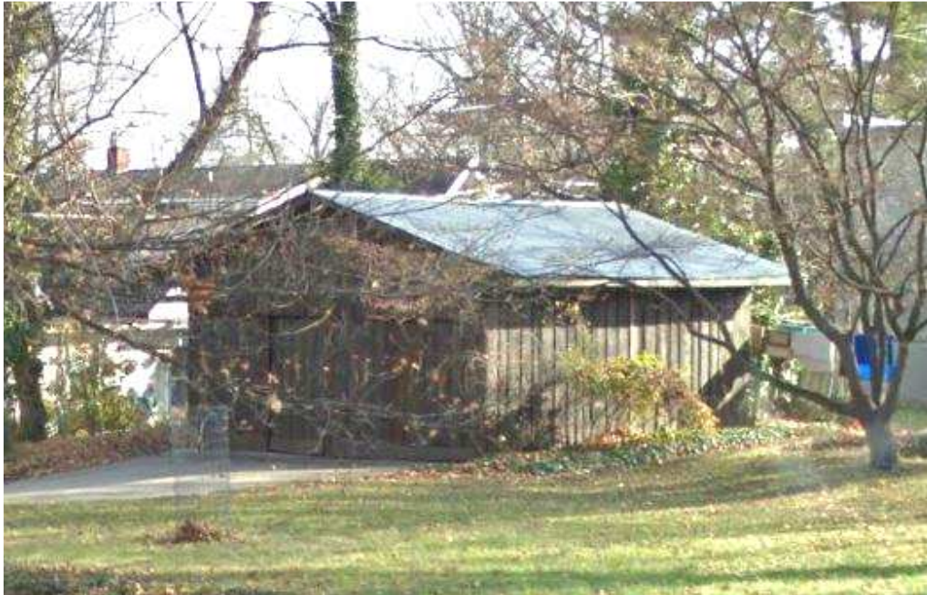
Figure 4: Non-contributing outbuilding on property. Source: Google maps, accessed April 2015.
