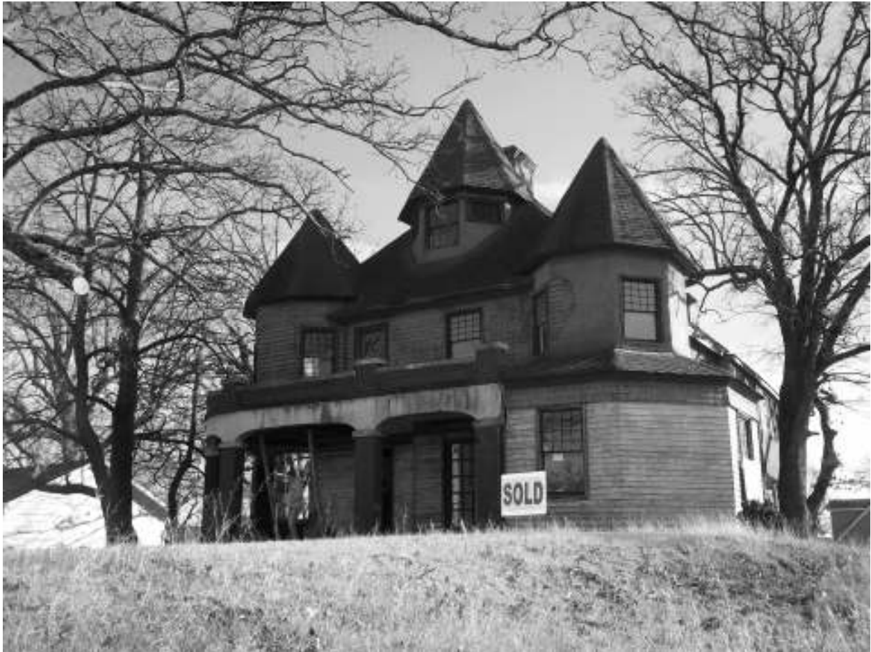
Figure 5: Photo of house prior to restoration.
