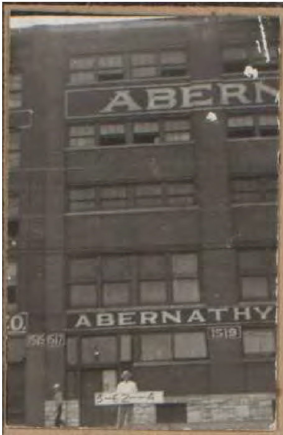
Figure 13: Abernathy Furniture Co., 1517-21 W. 9 th St., north elevation, 1940. Source: Missouri Valley Special Collections, Kansas City Public Library, Kansas City, Missouri.
