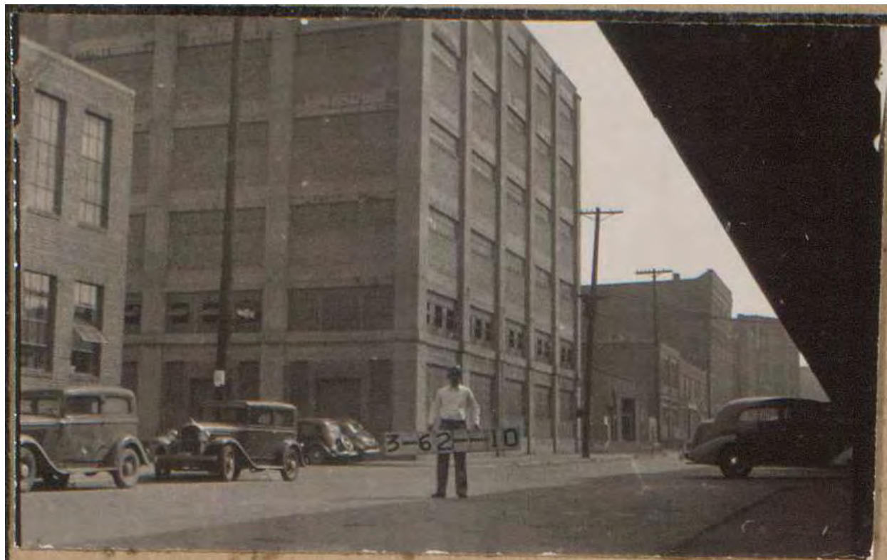
Figure 19: Hogue Mercantile Co. (left), 1600-02 St. Louis Ave., and Bemis Bros. Bag Co., 937 Wyoming St., looking northeast, 1940. Source: Missouri Valley Special Collections, Kansas City Public Library, Kansas City, Missouri.
