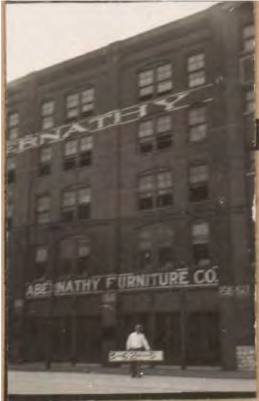
Figure 12: Abernathy Furniture Co., 1511-15 W. 9 th St., north elevation, 1940. Source: Missouri Valley Special Collections, Kansas City Public Library, Kansas City, Missouri.
