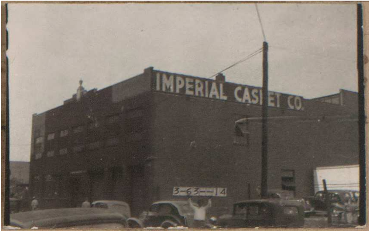
Figure 18: Imperial Casket Co., 920-24 Wyoming St., east and north elevations, 1940. Source: Missouri Valley Special Collections, Kansas City Public Library, Kansas City, Missouri.
