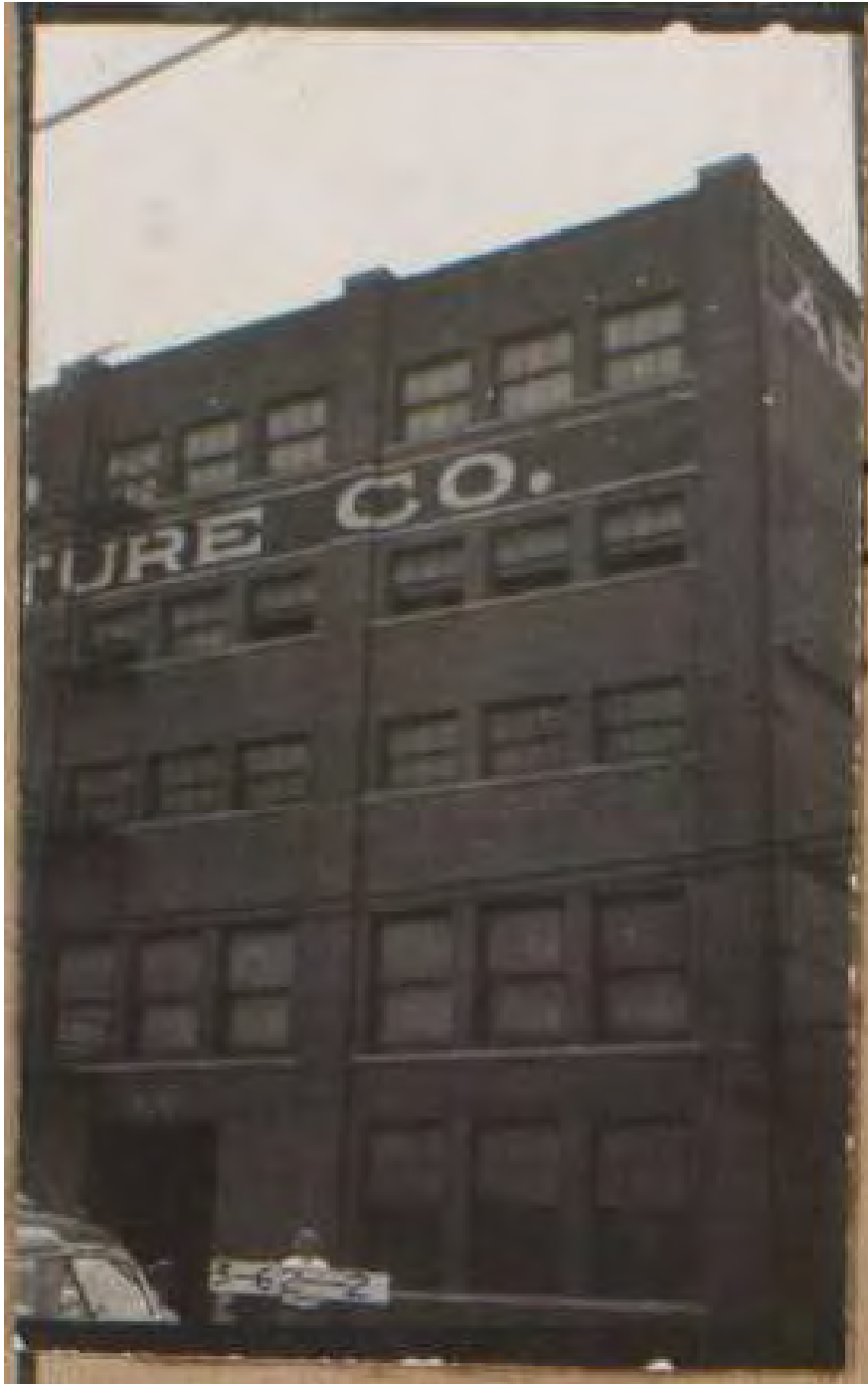
Figure 16: Abernathy Furniture Co., 1523-27 W. 9 th St., north elevation, 1940. Source: Missouri Valley Special Collections, Kansas City Public Library, Kansas City, Missouri.
