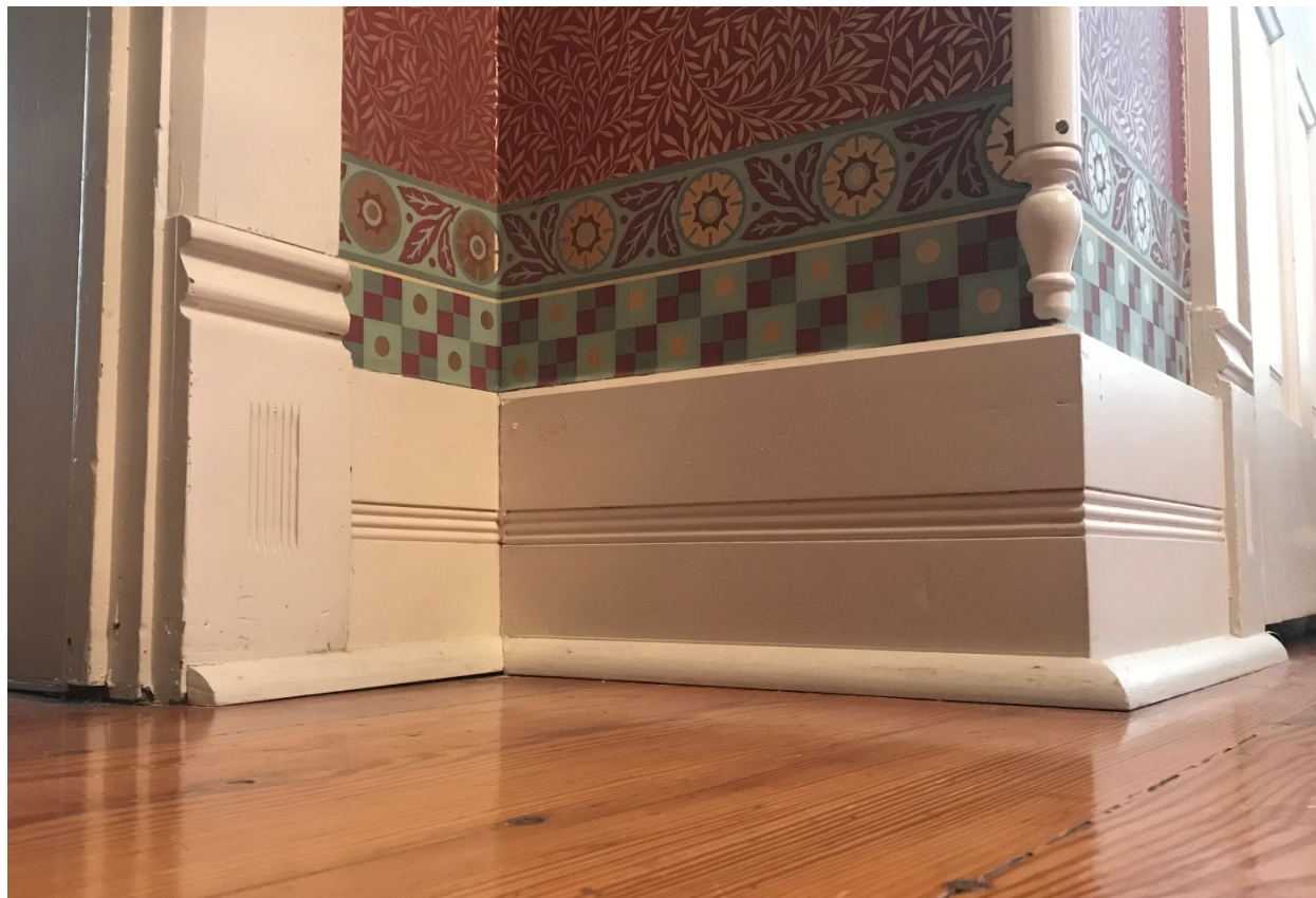
Figure 12: Typical Second Floor Trim, Baseboard and Door.
