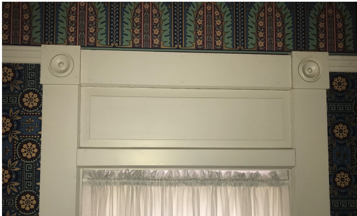
Figure 13: Typical Second Floor Trim, Door and Picture Rail.
