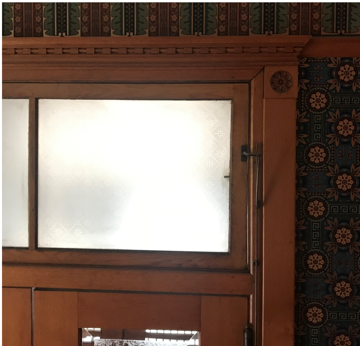
Figure 11: Typical First Floor Trim, Door and Picture Rail.
