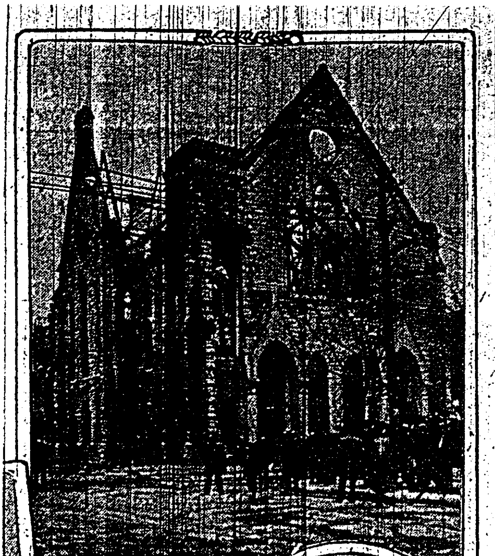
Figure 1: Exterior of Union Methodist Church after fire, from Post-Dispatch May 3, 1911.
