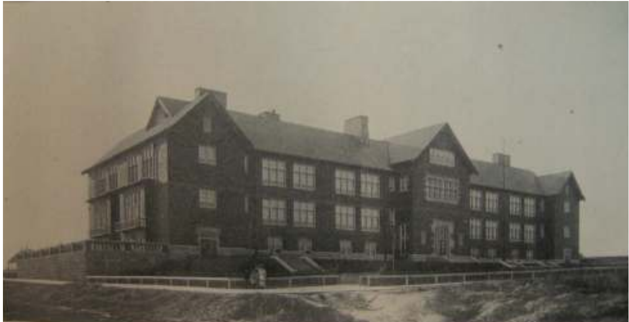
Figure 1. Historic Photograph, c. 1910
