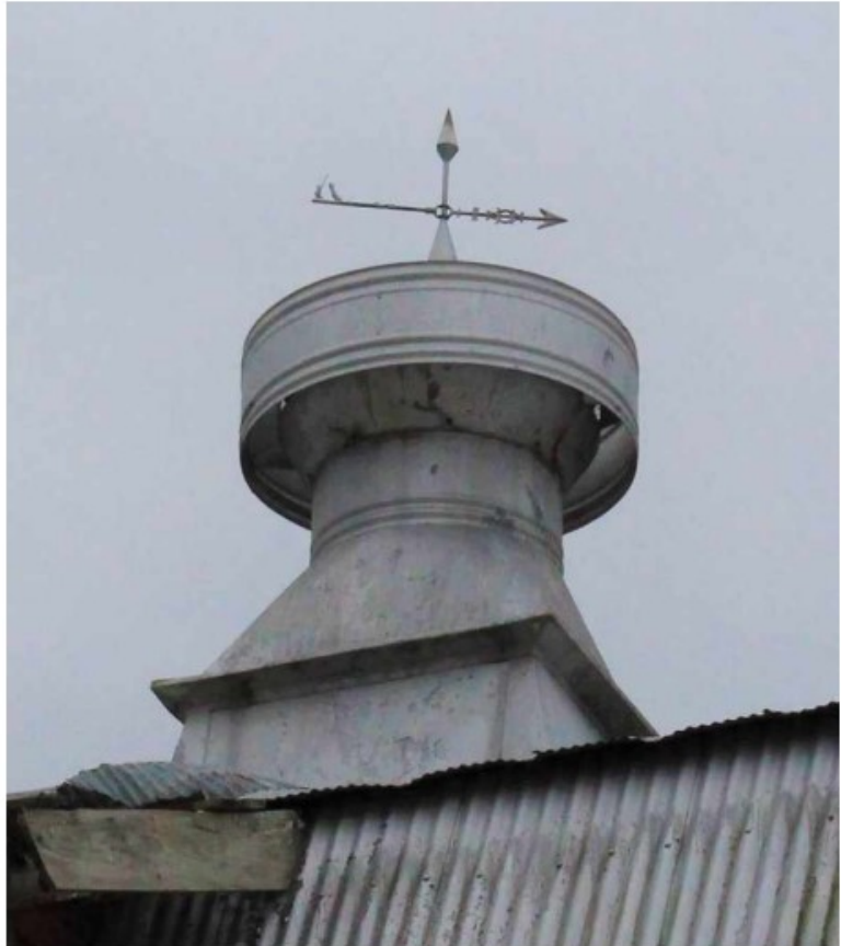
Figure 25. Comparison between the “James Flaring Base Ventilator,” (left) and a ventilator found on the Waggener Dairy Barn (right). ( Complete System of Jamesway Ventilation , Ft. Atkinson, WI: James Manufacturing Company, 1921, 20.)
