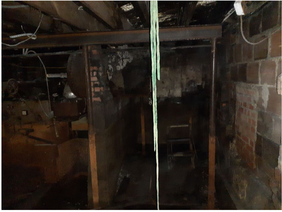
Figure 23: Basement (Former Dressing Room), facing north
