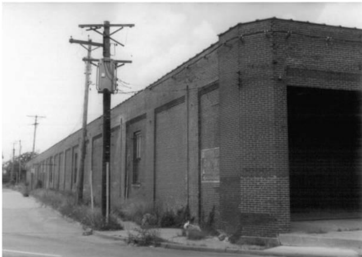
Figure 13. DeHodiamont Car Sheds, Landmarks Association of St. Louis
