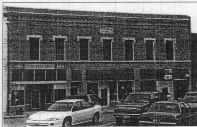
Figure 21: Bixler Block, 108-104 South 17 th Street, view northwest (photo by Jim Jacobsen, August 2001)
