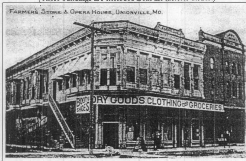
Figure 56: Northeast corner, 16 th and Main streets. These buildings burned in 1928
