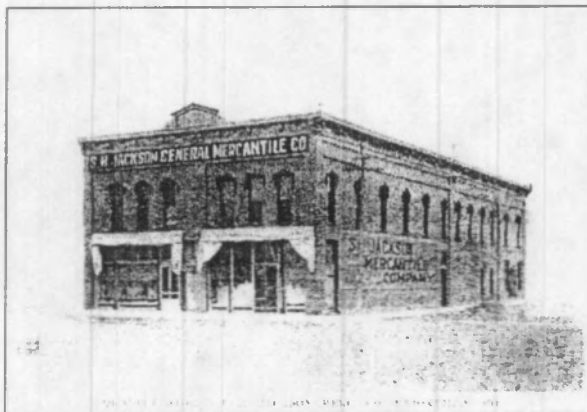
Figure 23: Doubled storefront, view southwest The single-story rear addition depicted in 1877 has become a two-story extension. Note pediment.
