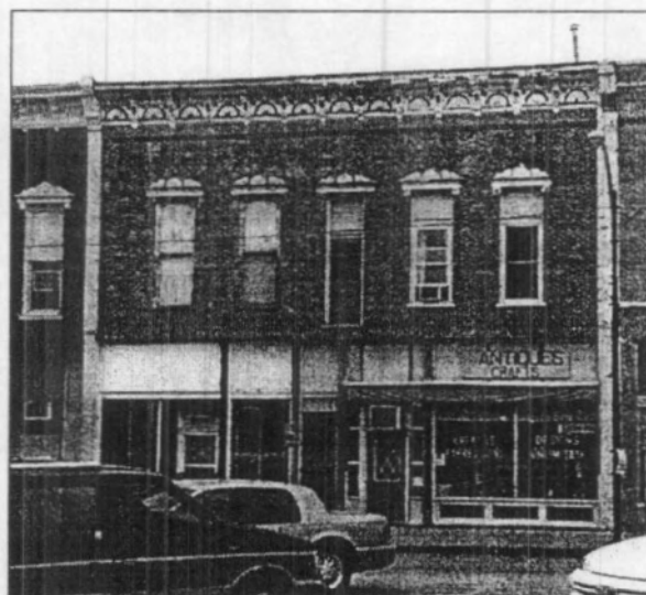
Figure 20: 112-110 South 17 th Street, view west (photo by Jim Jacobsen, August 2001)
