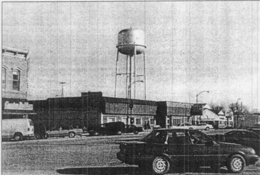
Figure 55: North side of square and northeast corner, view northeast (photo by Jim Jacobsen, December 2001) (These buildings are excluded from the historic district)
