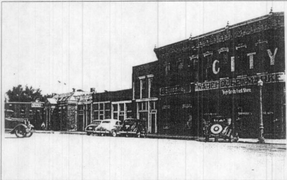
Figure 63: Same as previous, view to the southeast, 1940
