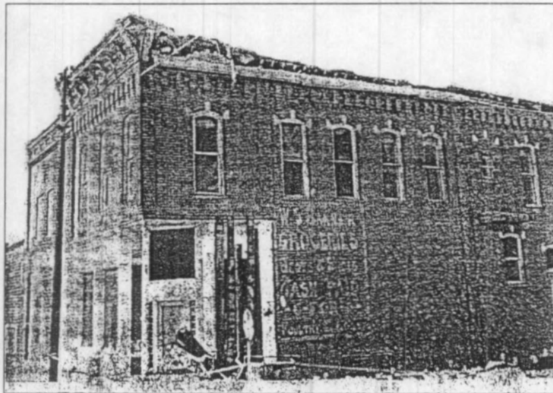
Figure 16: Remodeling 200 South 17 th Street, 1972, view southwest ( Unionville Republican , April 26, 1972)
