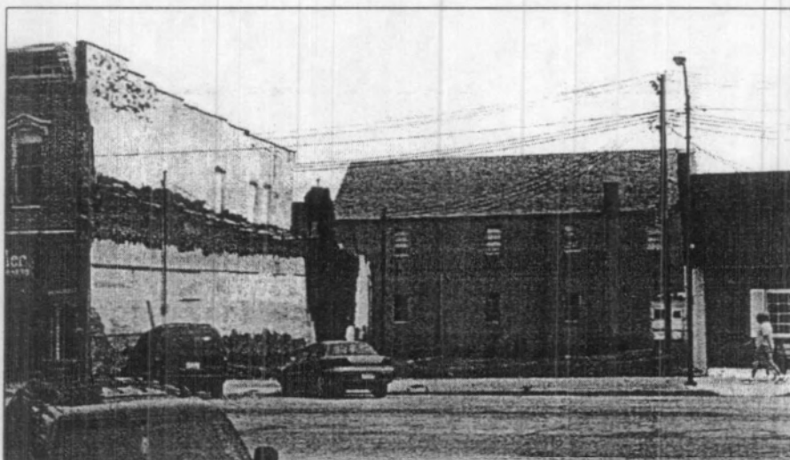
Figure 25: Gable roof portion of 116 N. 17 th Street, view north (photo by Jim Jacobsen, August 2001)
