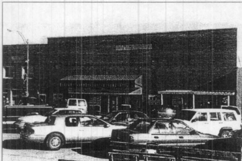
Figure 9: 117-117 South 16 th Street, view northeast (photo by Jim Jacobsen, December 2001)
