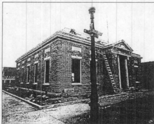
Figure 11: Construction photograph, December 2, 1931, view southwest (Post office archives)
