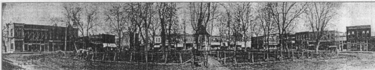
Figure 43: Panoramic view, view northwest, November 16, 1908, photo by M. E. Dye (Library of Congress)
