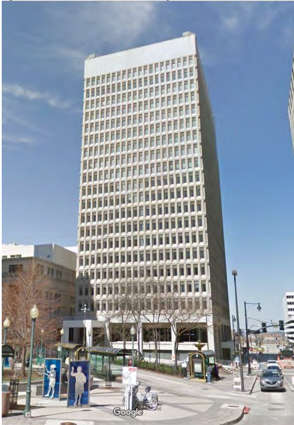
Figure 23. Ten Main Center, 2015. Source: Google Street View.
