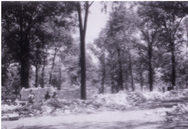
Figure 14. W.P.A. photo of Tilles Park under construction, ca. 1935 (source of photographs unknown, copies held by St. Louis County Parks and Recreation Department).
