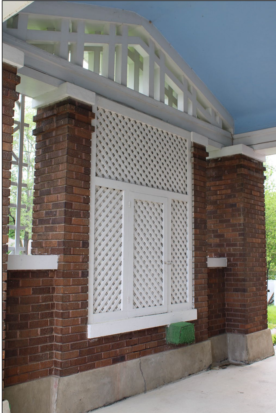
Figure 9: Detail of porte cochere with water well; view facing northwest, 2022.
