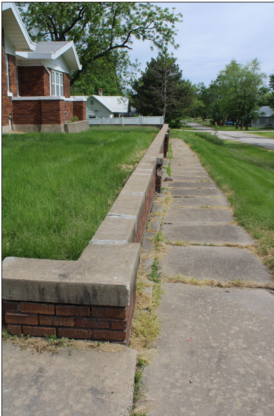
Figure 7: Detail of brick retaining wall with concrete cap; view facing north, 2022.
