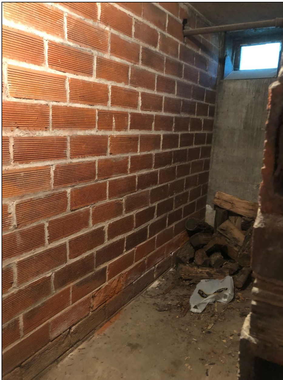
Figure 16: Basement level, wood storage room with chute to exterior; view facing southwest, 2022.
