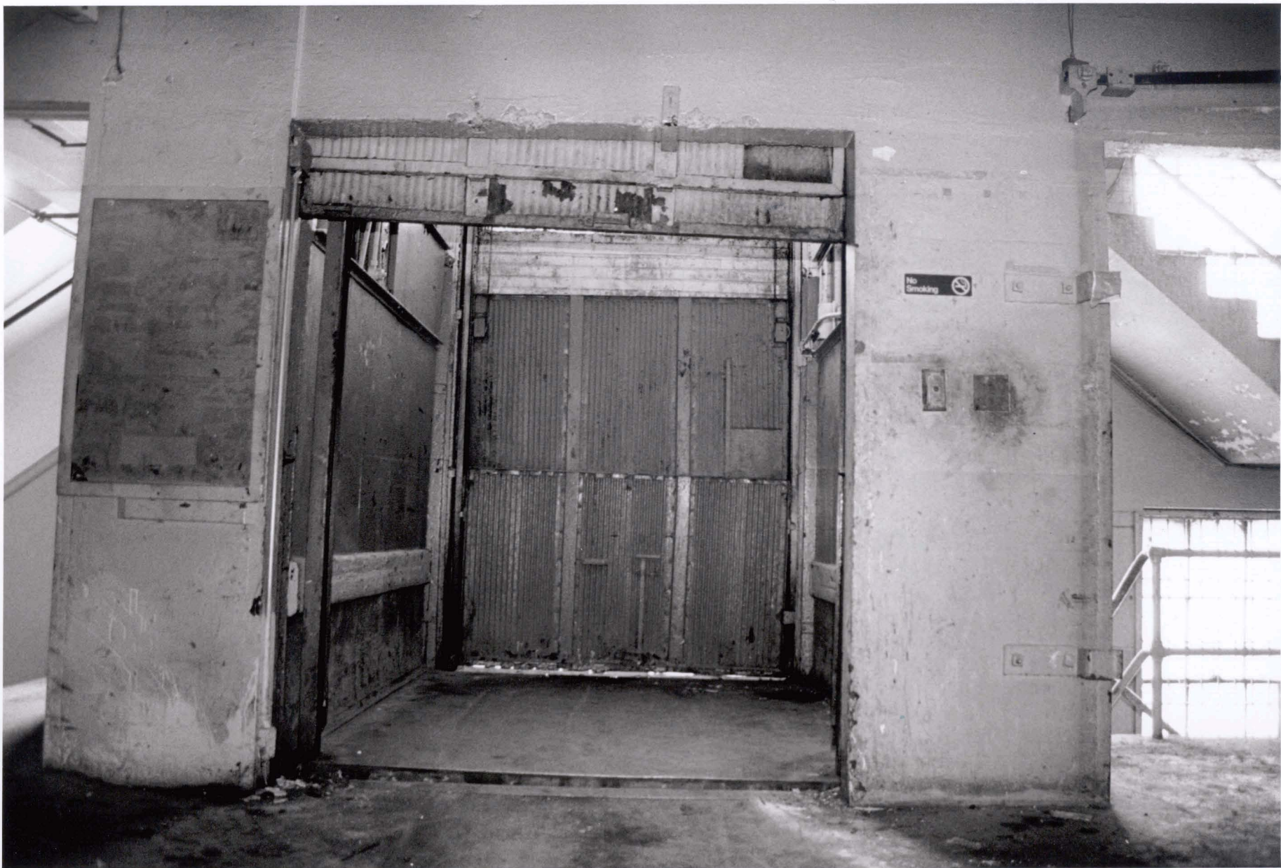
Steelcote Manufacturing Company Paint Factory St. Louis (Independent City), MO Photo # 8
