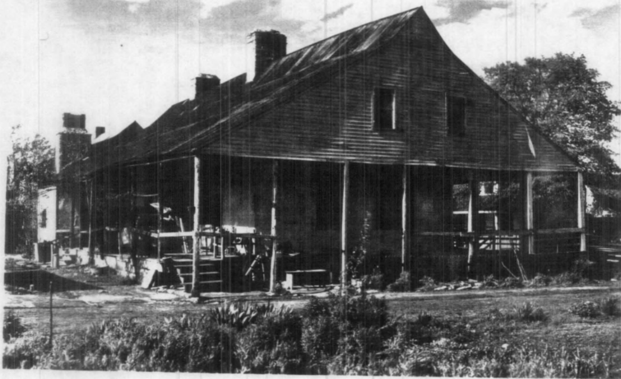
II - A. Bolduc House . General View, showing plastered poteaux sur sole walls and surrounding porch. Structure originally had hipped roof. Photograph by Charles E. Peterson.
