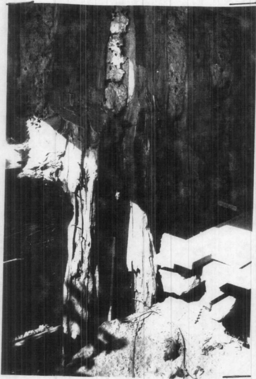
III - B. Ribault House . Detail of palisadoed or poteaux en terre construction. Cedar logs bougillé with clay and grass. Photograph by Charles E. Peterson.
