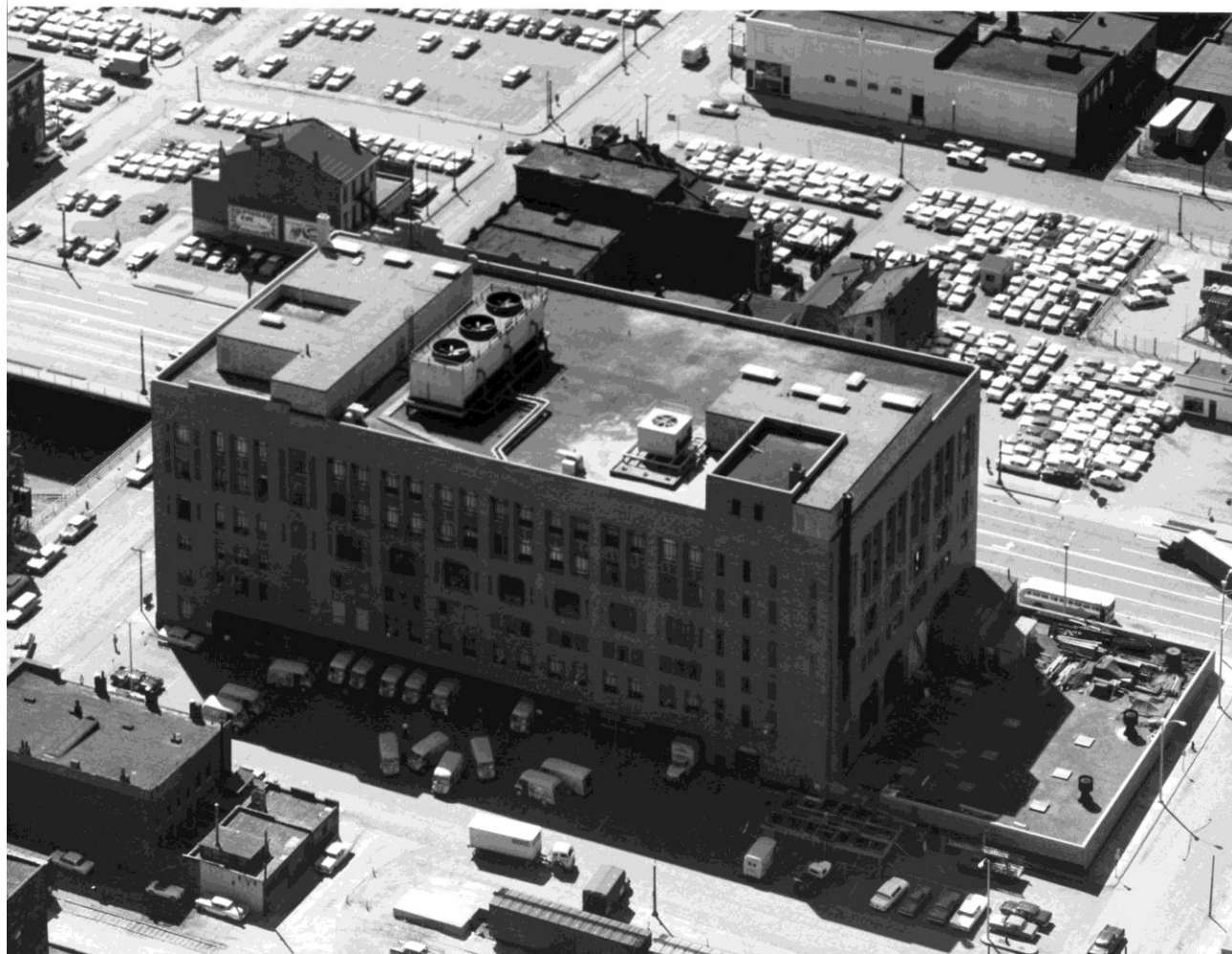
Post-Dispatch, - Bldgs. #9. Staff Photographer. Ferguson. Received by Post-Dispatch Reference Department April 30, 1982. Courtesy of St. Louis Post-Dispatch Photo Archives Reference Department. Aerial looking southwest at north and east elevations. Circa 1955.
