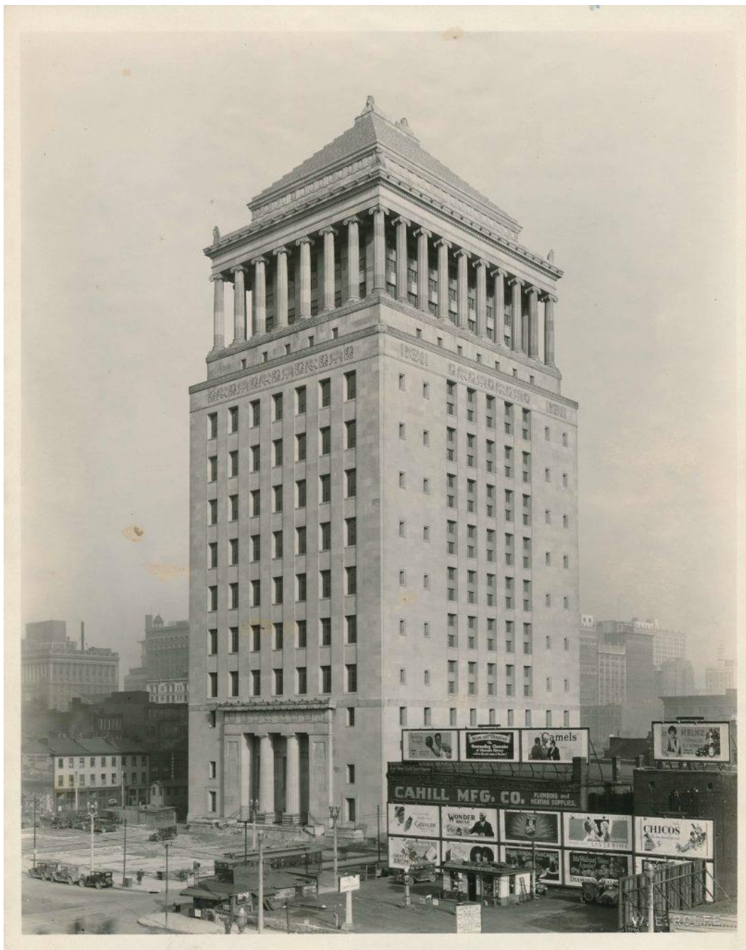
Civil Courts Building, c. 1930 (Source: National Building Arts Center, Available at: http://web.nationalbuildingarts.org/recovery-projects/courthouses/civil-courts-building/ , Access date: 26 September 2018).
