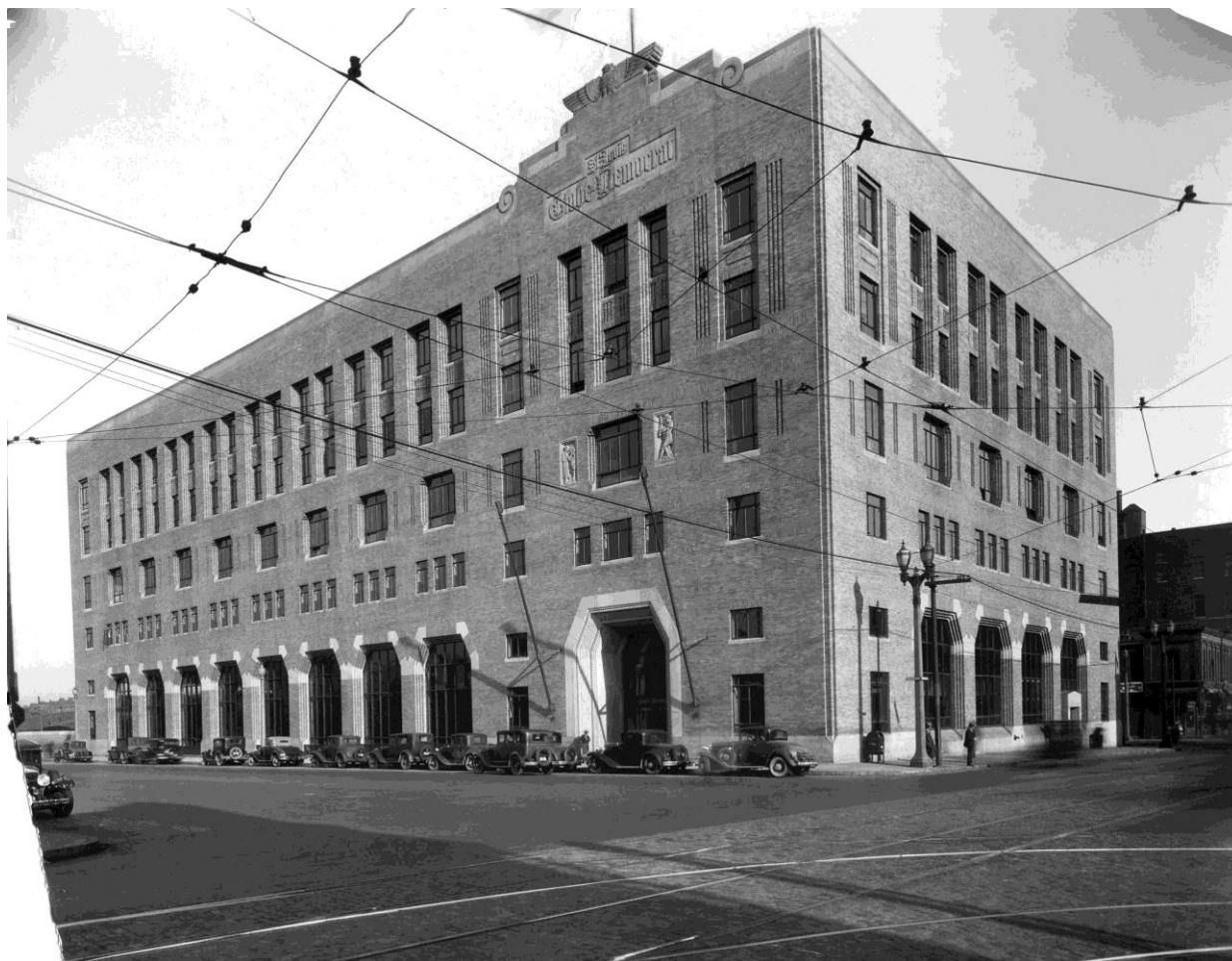
Post-Dispatch, - Bldgs. #9 (1133 Franklin) January 20, 1933. Courtesy of St. Louis Post-Dispatch Photo Archives Reference Department. Photo looking northeast at south and west elevations.
