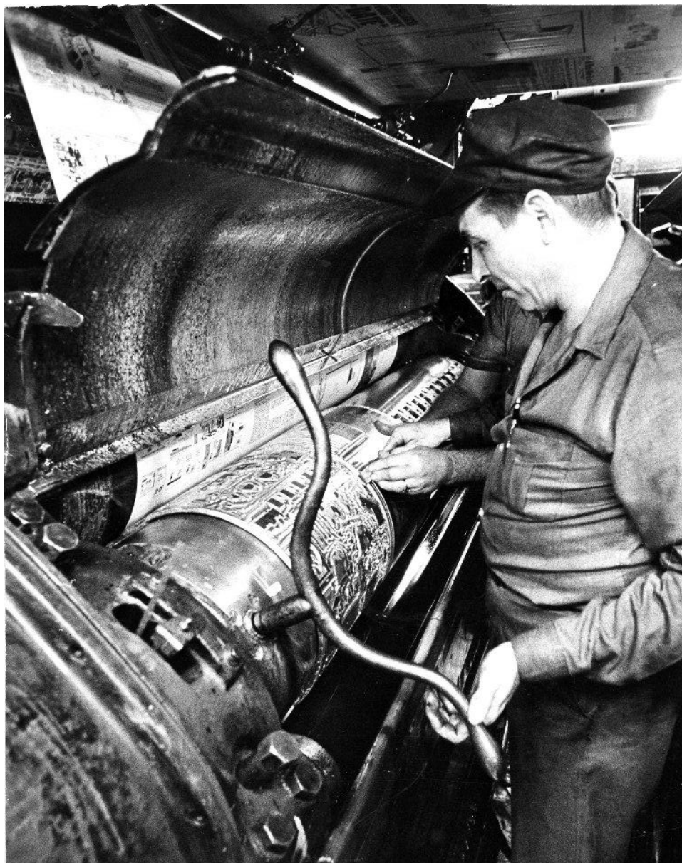
Post-Dispatch, - Bldgs. #9. April 25, 1973. Robert C. Holt III. Received by Post-Dispatch Reference Department April 28, 1973. Courtesy of St. Louis Post-Dispatch Photo Archives Reference Department. Photos taken as they were installing new presses and phasing out the linotype press.
