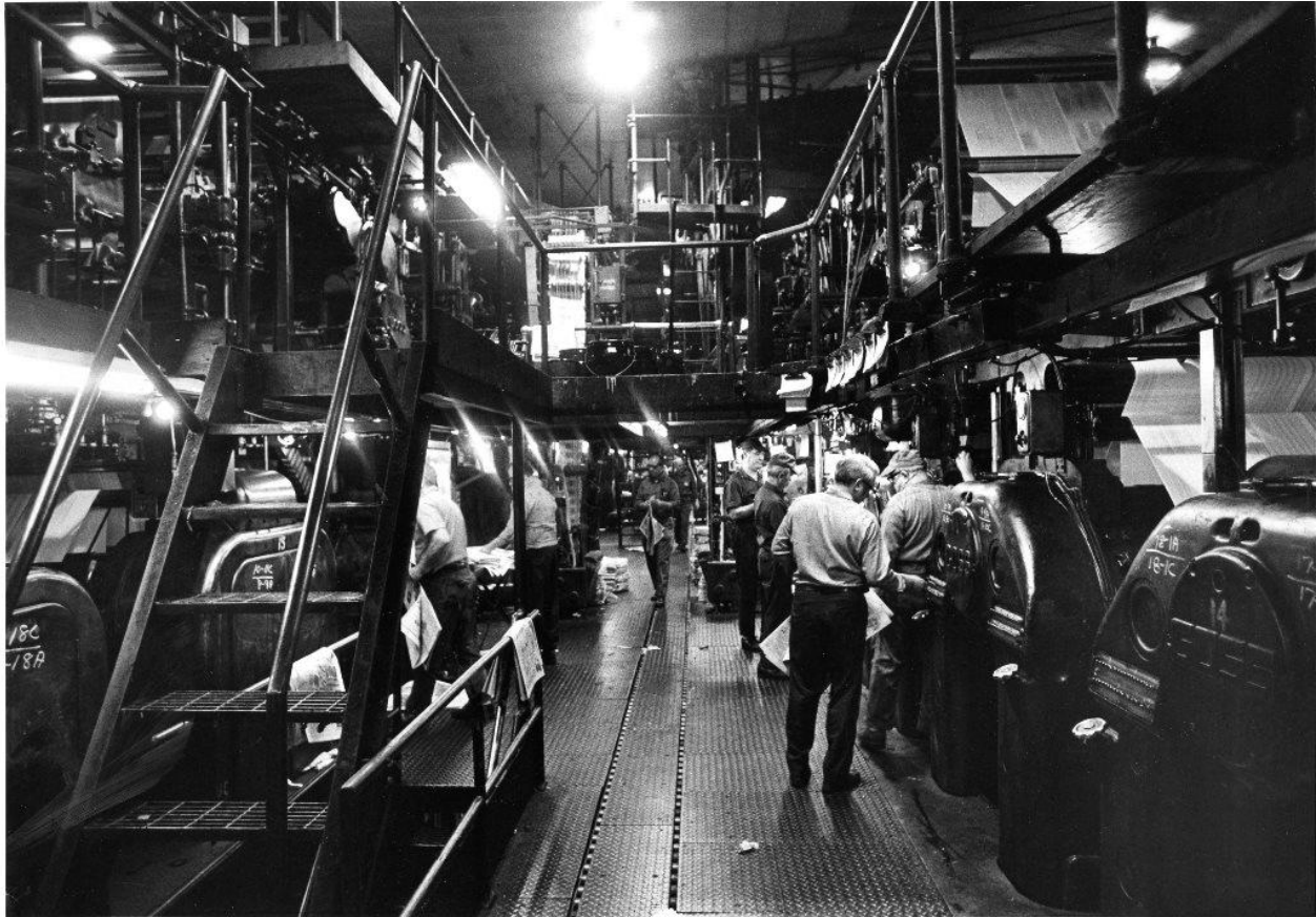
P.D. – BLDGS #9. December 5, 1972. January. Received by Post-Dispatch Reference Department. Courtesy of St. Louis Post-Dispatch Photo Archives Reference Department. Photos taken as they were installing new presses and phasing out the linotype press.
