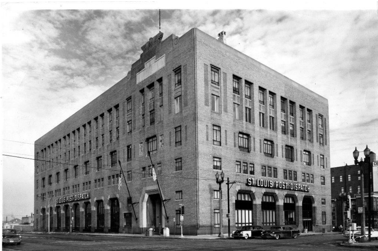
Post-Dispatch, - Bldgs. #9. 1133 Franklin. Received by Post-Dispatch Reference Department July 20, 1962. Courtesy of St. Louis Post-Dispatch Photo Archives Reference Department. Photo looking northeast at south and west elevations.
