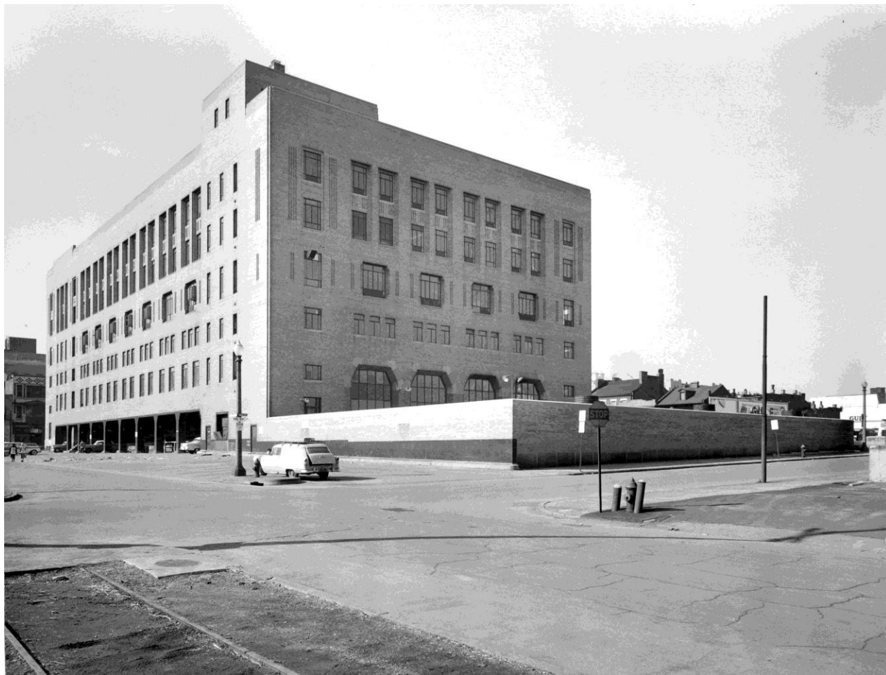
Post-Dispatch, - Bldgs. #9 (1133 Franklin) Received by Post-Dispatch Reference Department March 19, 1959. Courtesy of St. Louis Post-Dispatch Photo Archives Reference Department. Photo looking southwest at north and east elevations.
