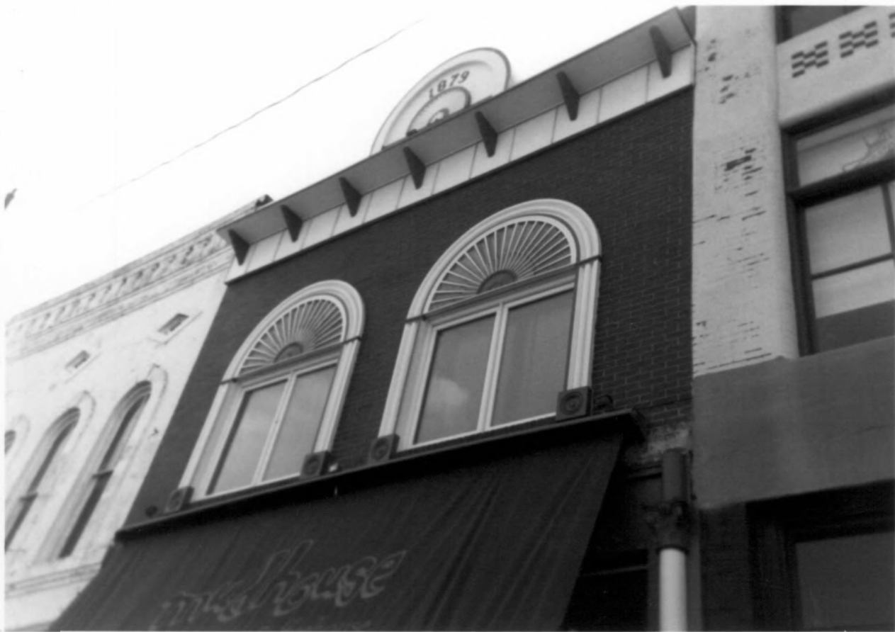
323 South Avenue Springfield, Greene Co., MO
