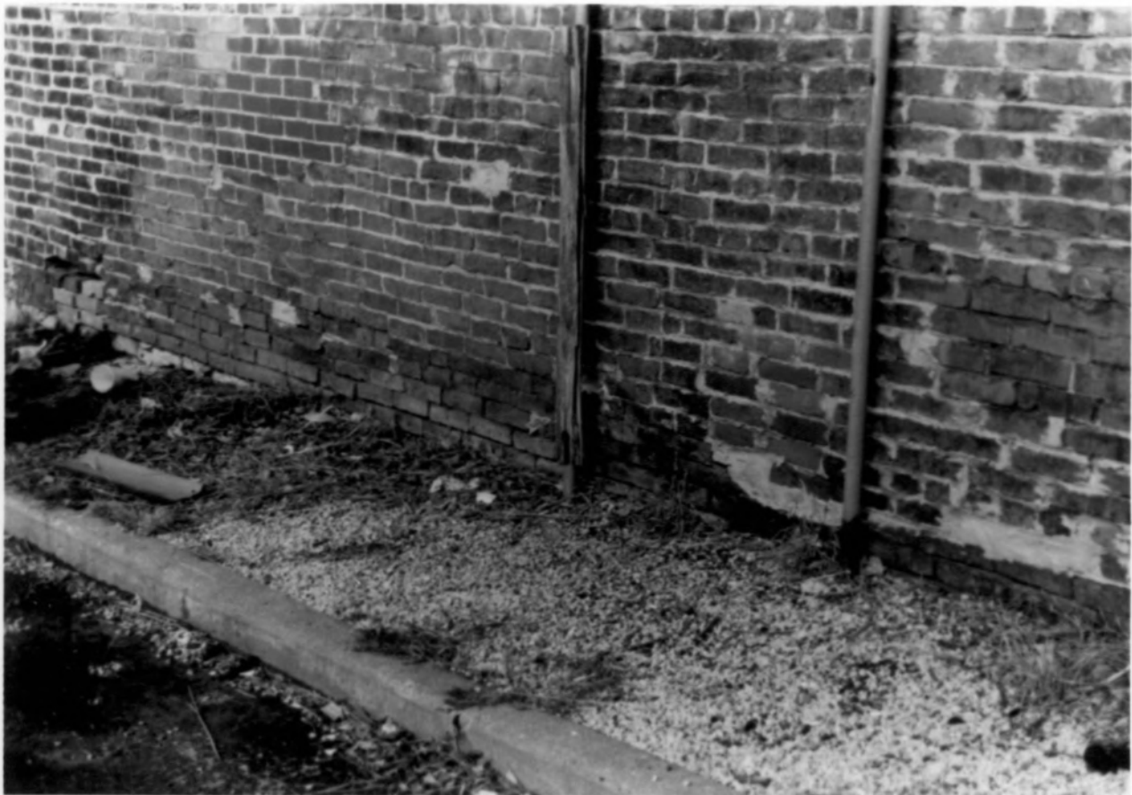
323 South Avenue Springfield, Greene Co., MO Prework Photo 5
