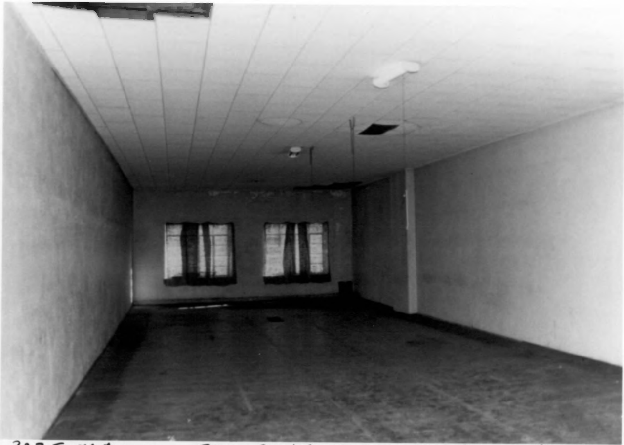
323 South Avenue Springfield, Greene Co., MO Prework Photo 7
