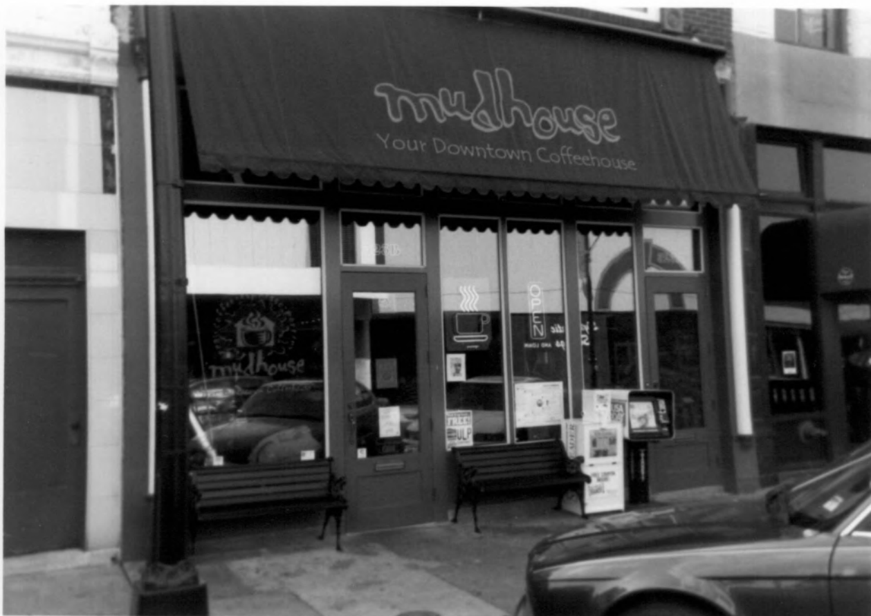
323 South Avenue Springfield, Greene Co., MO
