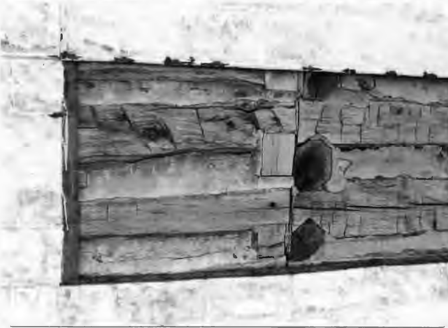
EXTERIOR DETAIL SHOWING NOTCHING AND METAL PANELS
