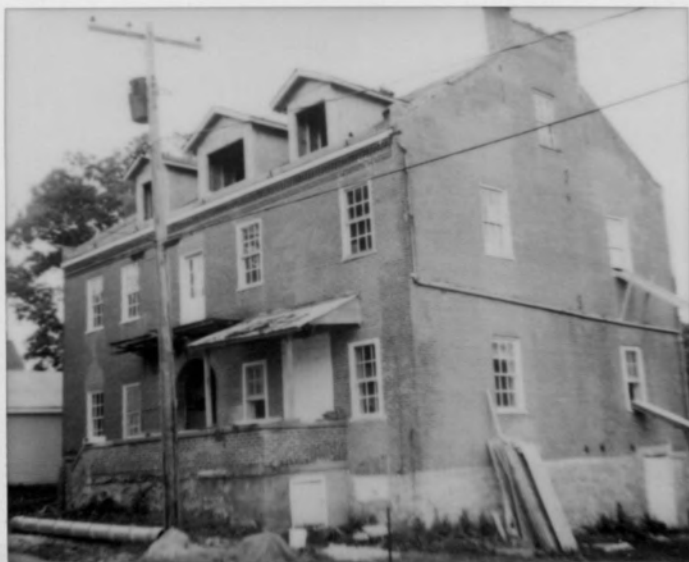
Schrow House/Himling Hotel after
