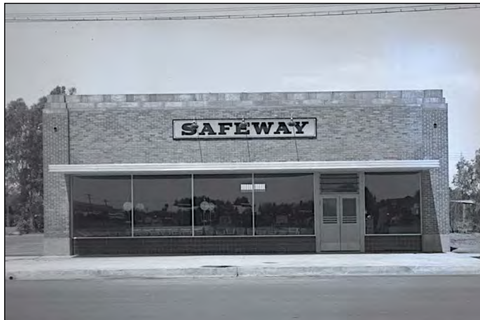
Figure 16: Safeway Streamline plan designs in Vancouver, Canada, c. 1940 (top) and Arizona, United States, 1942 (bottom).
