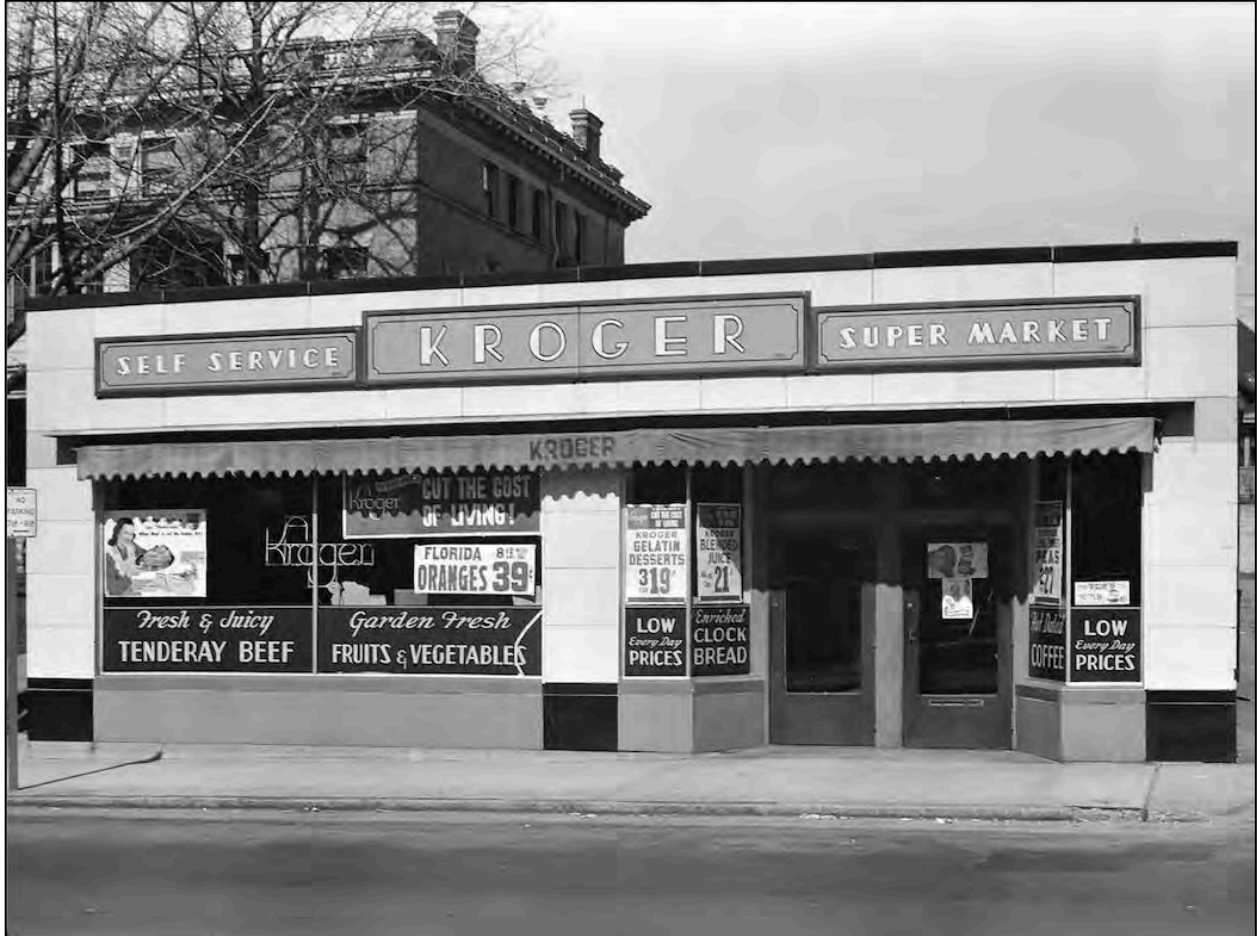
Figure 14: An example of a stand-alone grocery store, constructed c. 1930s, photo taken 1948.
