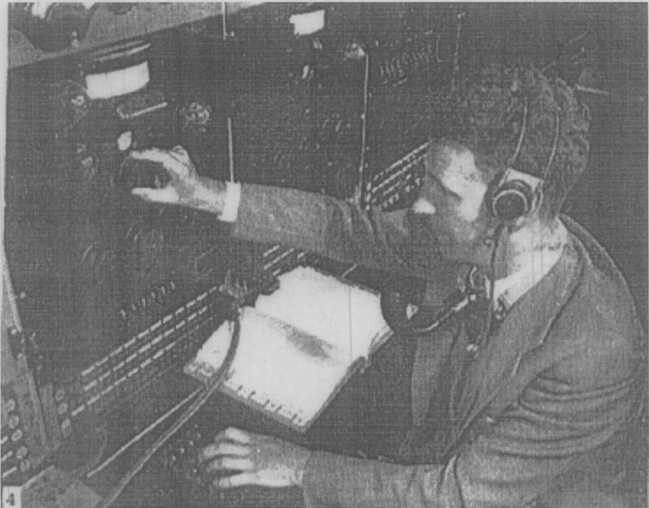
Figure 6: "A Camera Trip through a Repeater Station." August through September 1937. Step four. Source: AT&T Archives & History Center Collection, San Antonio, Texas.
