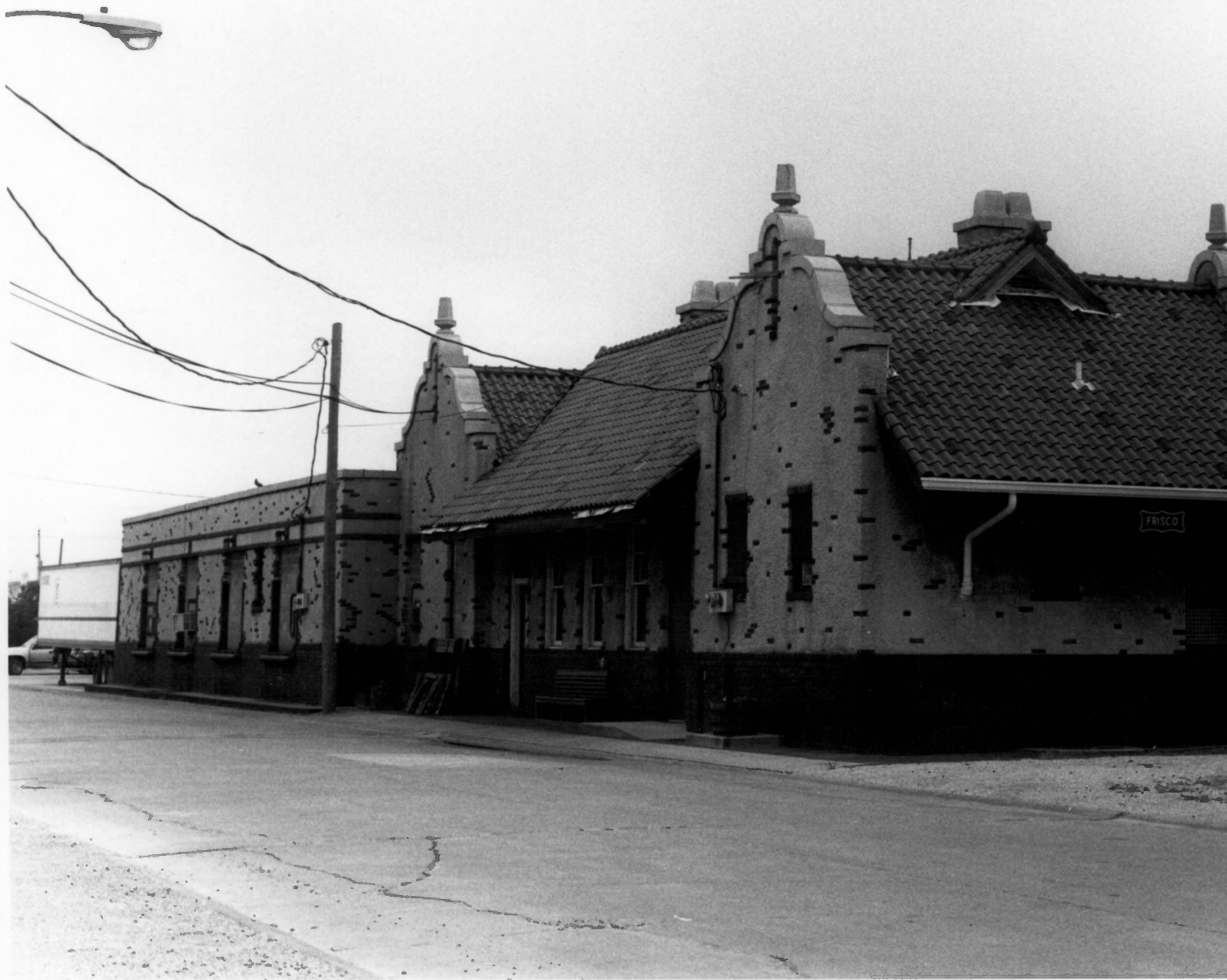
Photo # 1 of 4, Frisco Depot - 303 Moran St., Poplar Bluff, MO - Butler Co.
