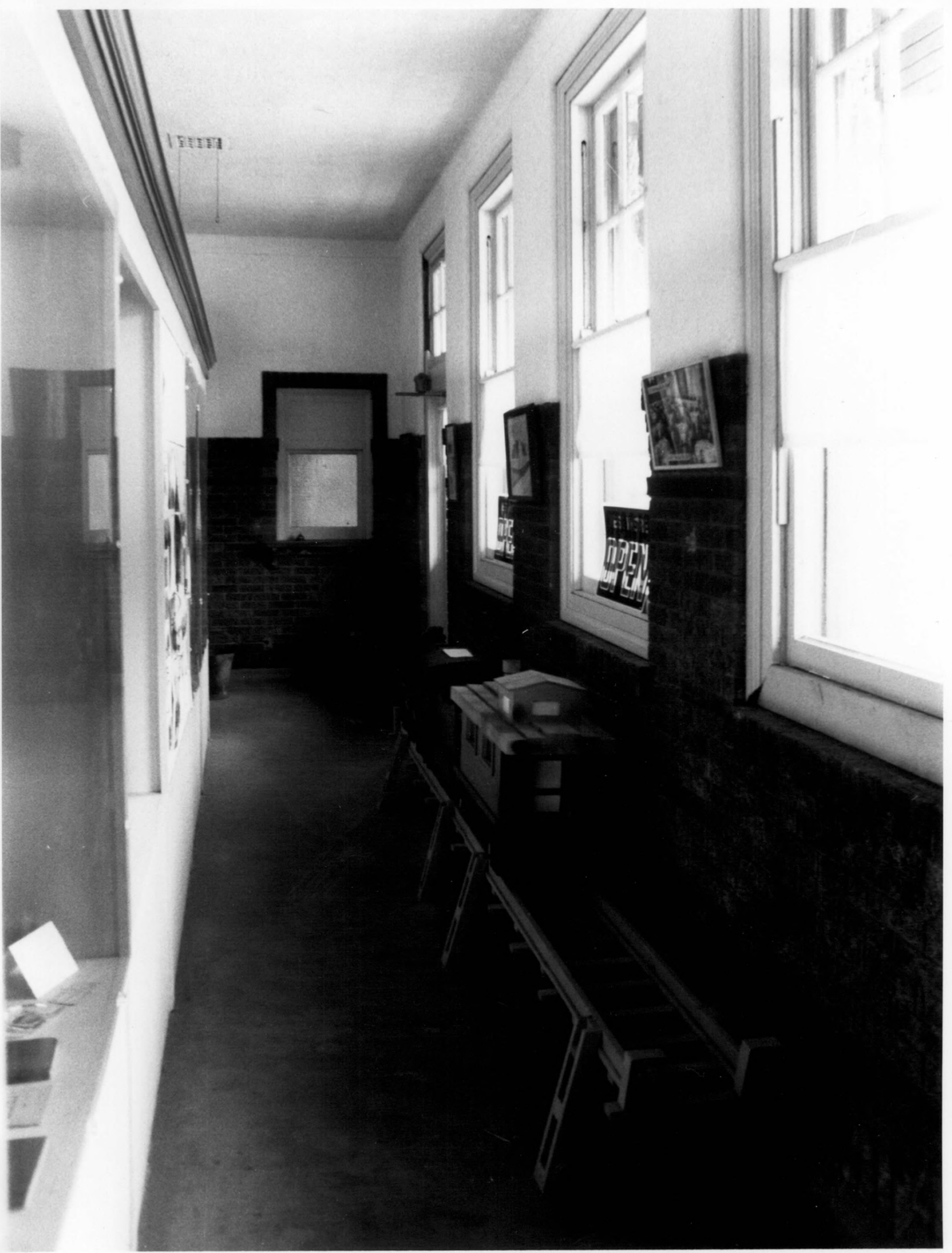
Photo #4 of 4, Frisco Depot - 303 Moran St., Poplar Bluff, MO - Butler Co.
