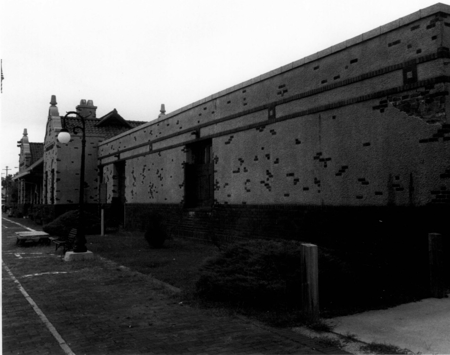
Photo # 3 of 4, Frisco Depot - 303 Moran St., Poplar Bluff, MO - Butler Co.
