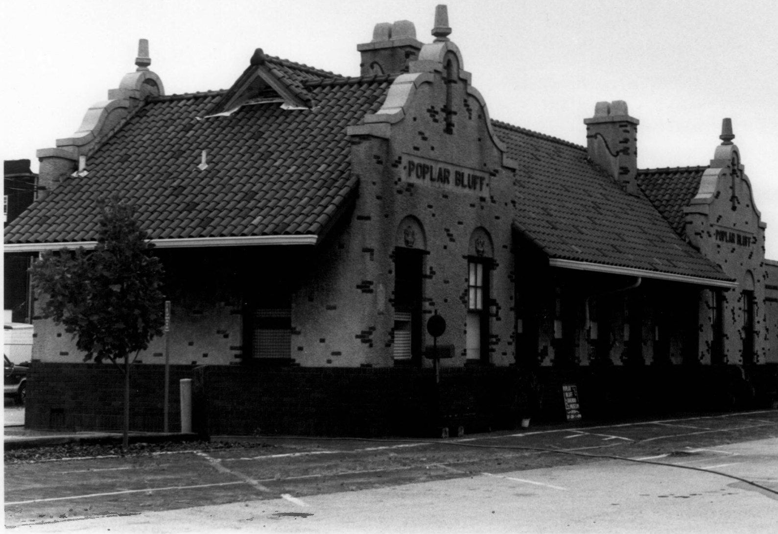
Photo # 2 of 4, Frisco Depot - 303 Moran St., Poplar Bluff, MO - Butler Co.
