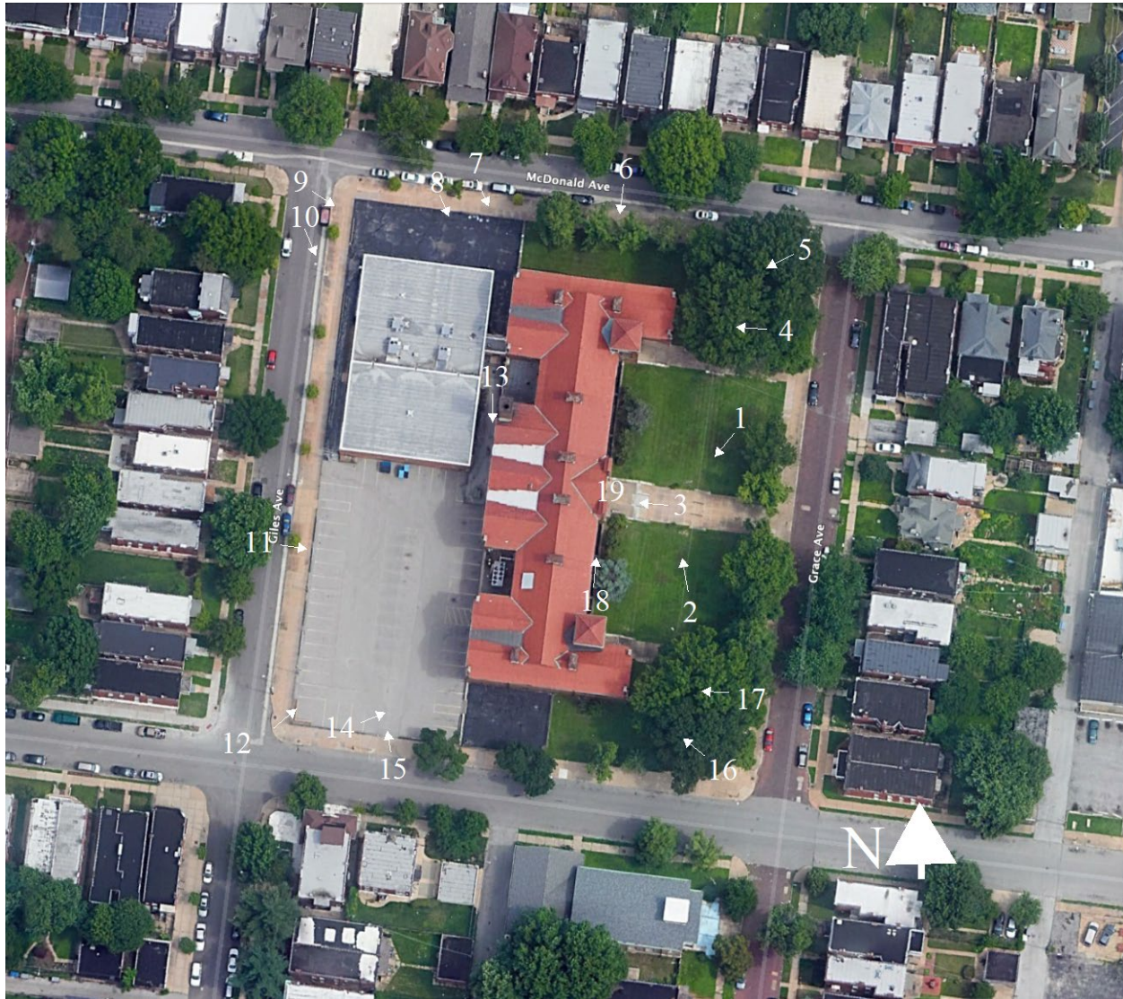
Figure 19. Exterior Photo Key (Aerial Image from Google Maps).
