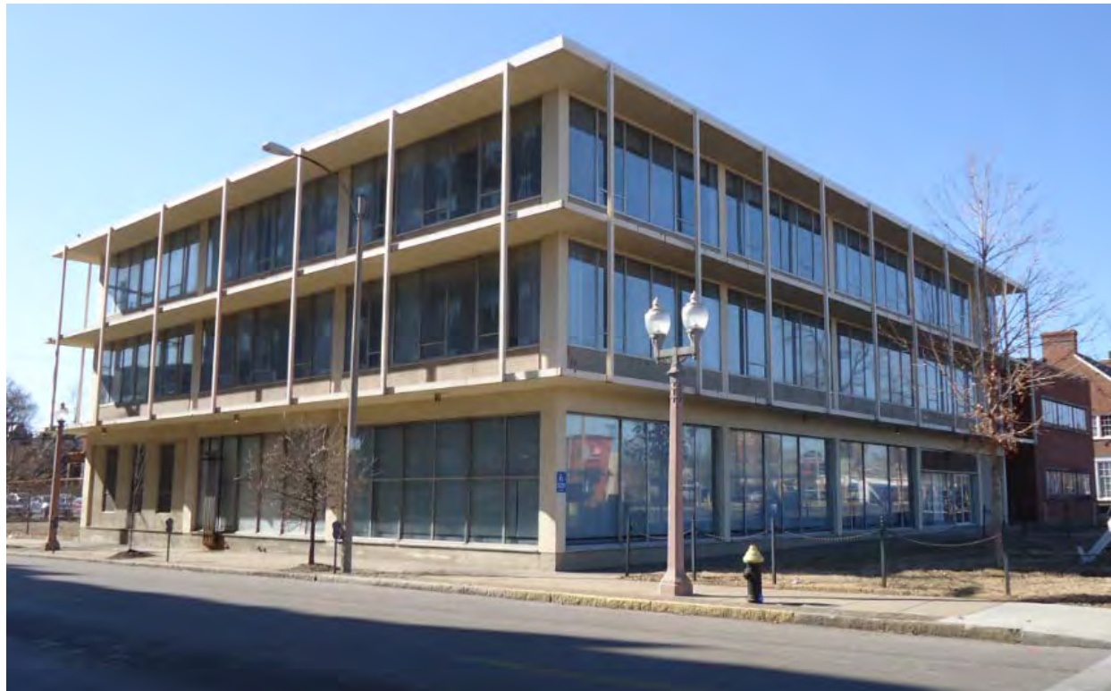
Figure 9: Remington Rand Building, built in 1956 at 4100 Lindell. Source: Matt Bivens photograph 2014.
