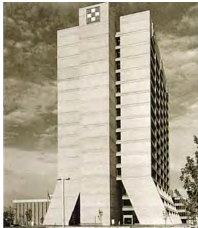
Figure 17: 1969 Ralston Purina Company, Checkerboard Square, St. Louis, Missouri. Source: "A Guide to the Architecture of St. Louis." George McCue and the Curators of the University of Missouri. (Columbia, Missouri: University of Missouri Press, 1989).
