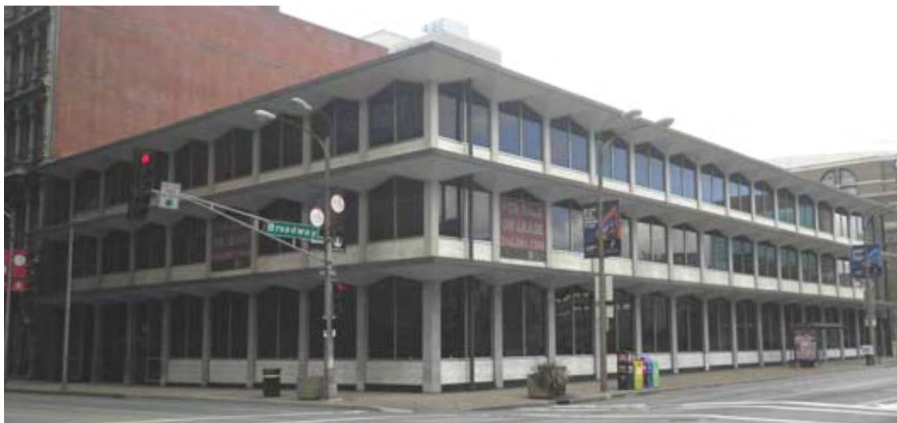
Figure 10: State of Missouri Office Building, built 1959 at 601 Broadway, St. Louis. Source: Google Earth, 2014.
