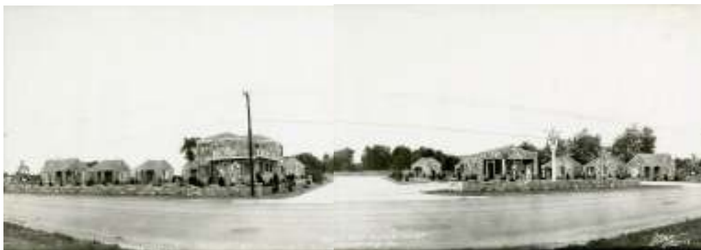
Figure 11: Historic Photograph. Trail's End Motor Court, Springfield, MO. Courtesy of the Historic Springfield Collection [M026], Department of Special Collections and Archives, Missouri State University (Springfield, MO).
