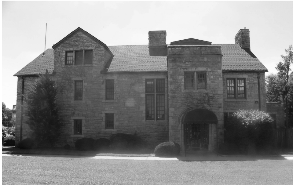
Figure 8: Photograph. Charles G. Martin House, Springfield, MO. Located at 1121 South Glenstone Avenue. It was acquired by Rex Rainey in 1952 as a possible site for a new funeral home business, but later sold. September 3, 2013. Richard Lee Burton.
