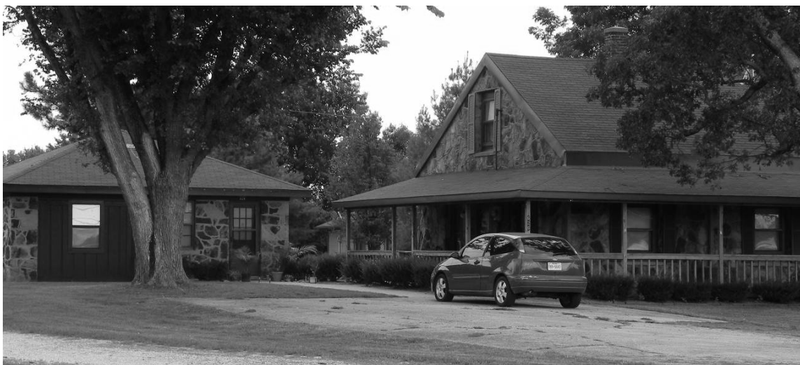
Figure 17: Photograph. Ozark Rock Masonry domestic dwelling, Marshfield, MO. Located at 540 South White Oak. August 16, 2013. Richard Lee Burton.
