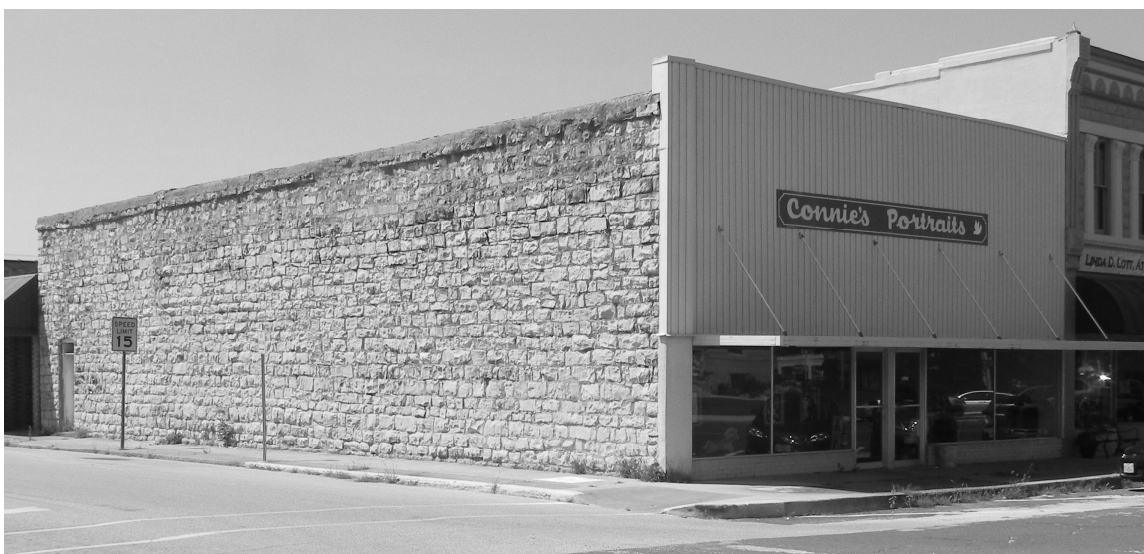
Figure 16: Photograph. Coarsed Rock Building, Marshfield, MO. Located at 108 East Madison Street. August 14, 2013. Richard Lee Burton.
