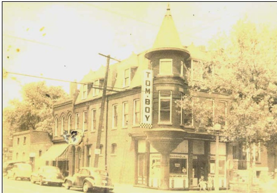
Figure 1. Front (South) façade and West Façade – circa 1948. (Photo from private collection of Anthony Garavaglia)
