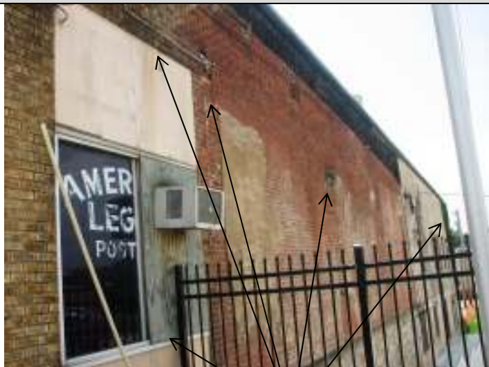
North elevation, showing crack in brick wall, boarded window, mortar issues, and vegetation on wall surface
