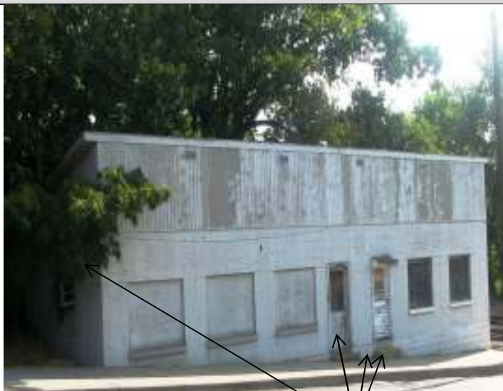
Façade, showing missing step, crack in foundation, deteriorated doors and overgrown vegetation
