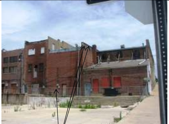
West and south elevation, showing leaning parapet wall, brick work issues, and graffiti
