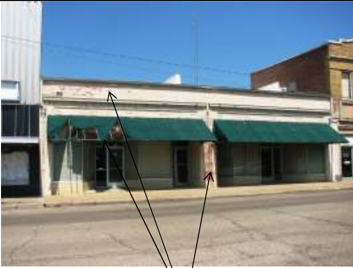
Façade (east), showing peeling paint, torn awning cover
