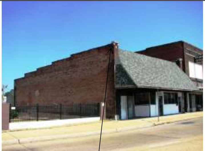
South elevation, showing loose brick
