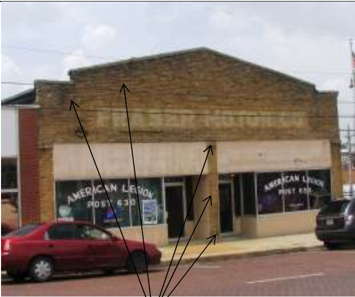
Façade, showing mortar issues
