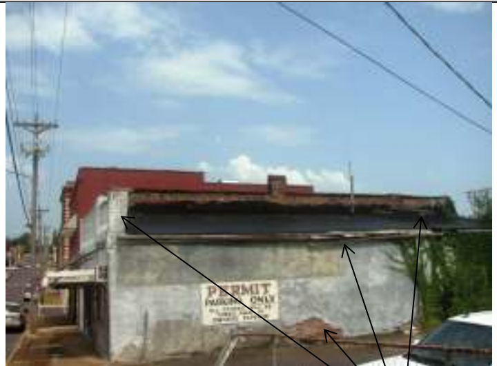
East elevation, showing missing stucco, leaning parapet, sagging roof, loose gutter, and cracks in brick roof ridge
