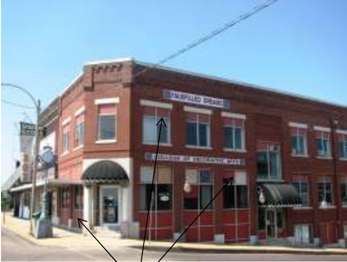
Façade (east) and north elevation, showing covered over windows
