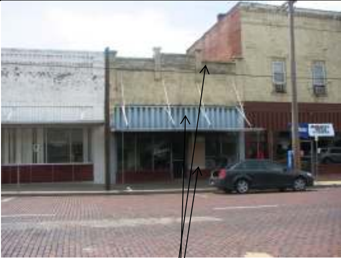
Façade (east), showing smoke damage on brick wall surface and awning, and missing store front window
