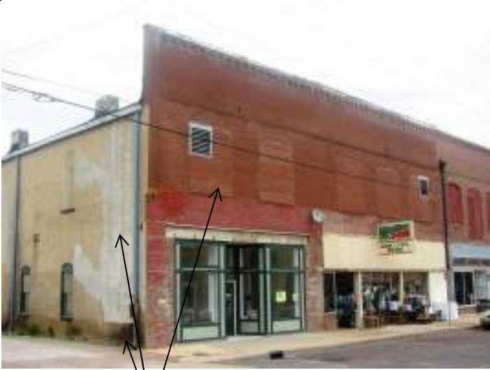
Façade (south) and west elevations – 415 is storefront on the left (end) – showing brick infilled windows, and deteriorated stucco. Water damage on lower section of west elevation
