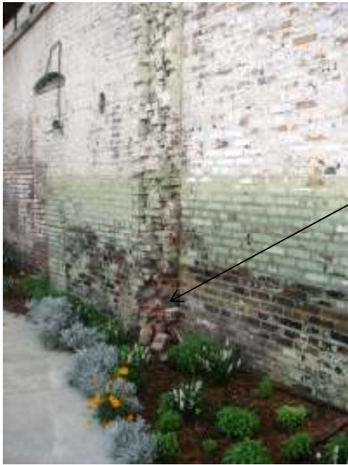
West elevation, showing fallen and loose bricks
