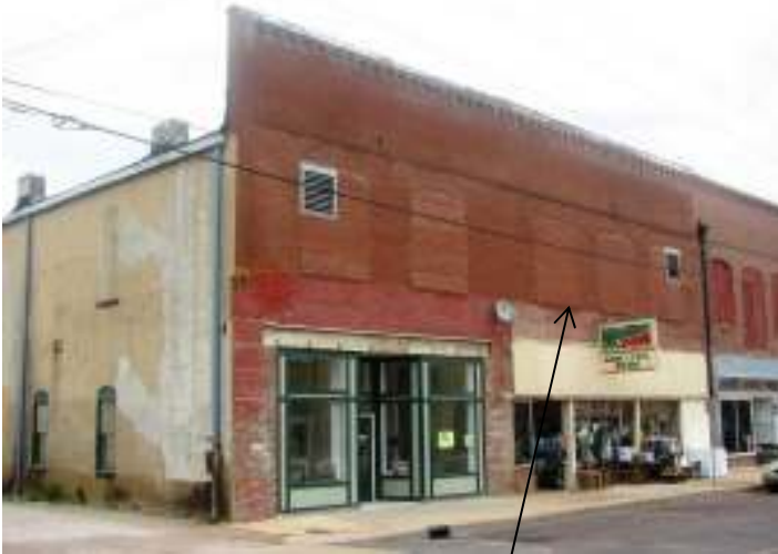
Façade (south) – 413 is second storefront from corner. Showing brick infilled windows
