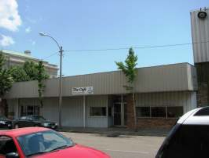
Façade (west) showing weathered metal siding
