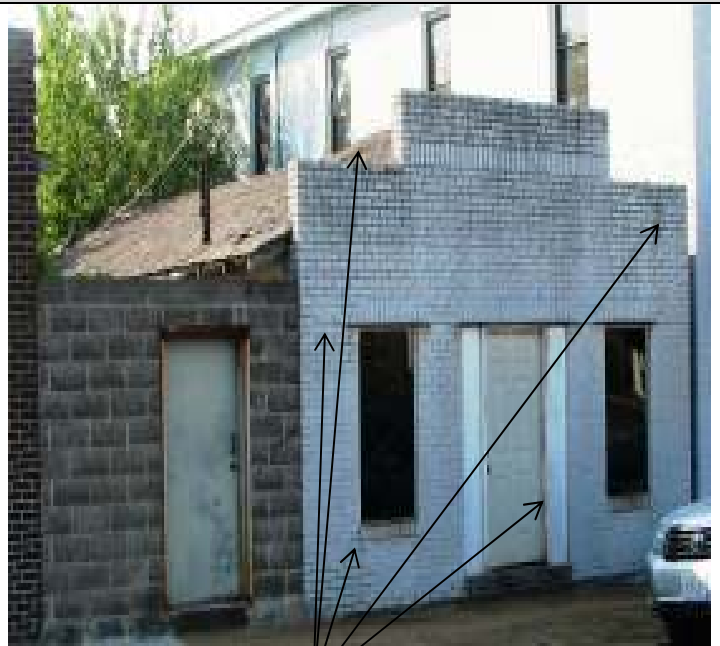
Façade (west) and north elevation, showing worn roof, deteriorated rafters, missing mortar, cracked brick, and weather door surround
