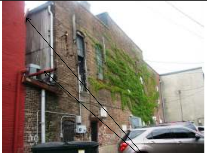
Rear (north) elevation – showing the west corner and disconnected downspout. Building is the red building in the photograph
