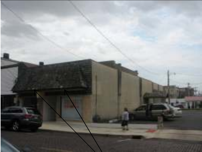
Facade (north), showing missing wood shingles
