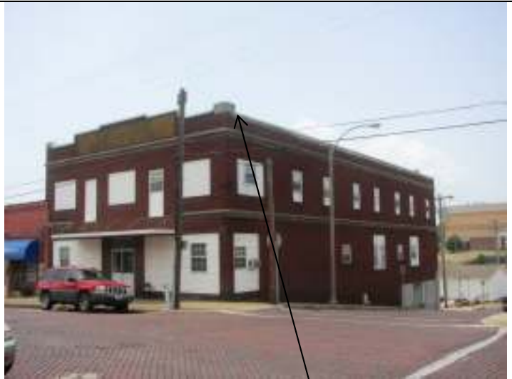
Façade and north elevation, showing improper re-pointing of brick and infill of windows
