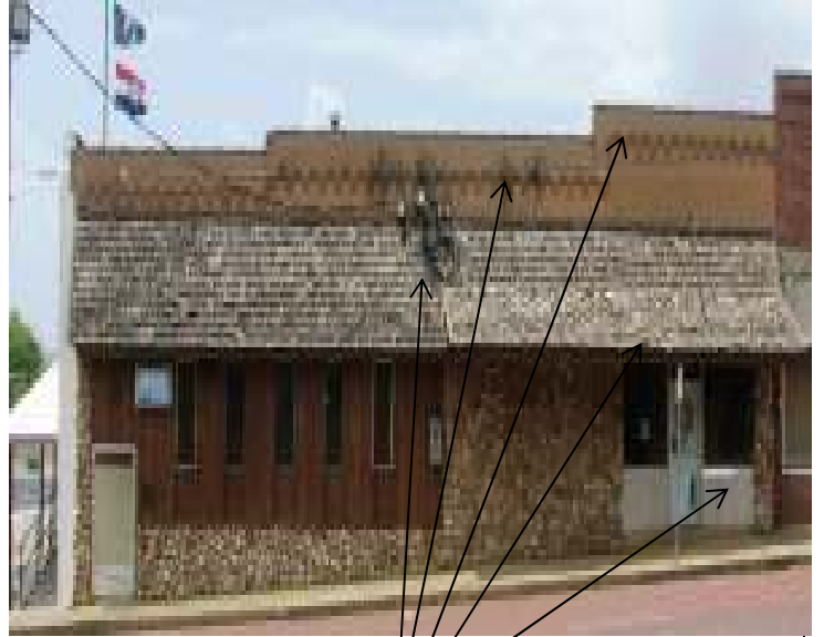
Façade, showing dent in bulkhead, loose/missing shingles, discolored bricks, wires/cables and cracks in brick wall surface.
