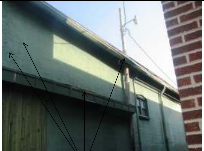
East elevation, showing bent gutter, deteriorated trim, and cracked brick wall surface
