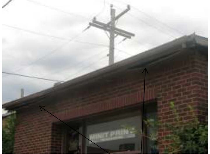
Façade, showing loose trim on the northeast and northwest corner of roofline
