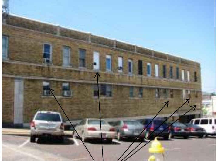
North elevation, showing boarded up windows, and missing windows, and vacant sign frame
