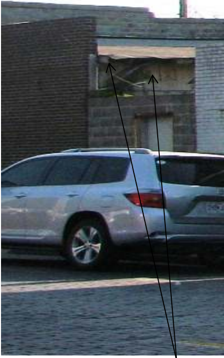
South elevation, showing the deterioration of the expose roof rafters and wall surface
