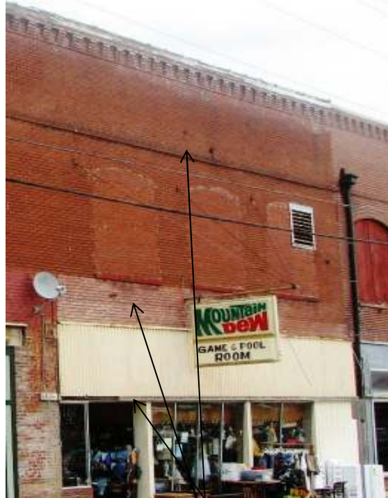
Façade – showing cracks in mortar, missing trim from metal slip cover and mortar issues
