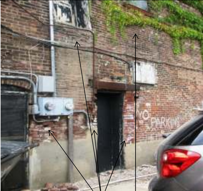
Rear (north) elevation, showing loose and fallen bricks, mortar issues, and vegetation on wall surface.
