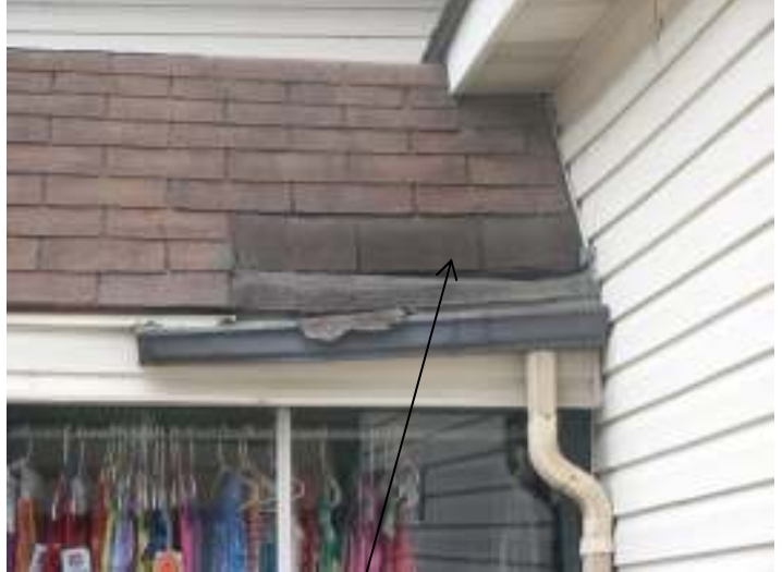
Façade; showing damaged roof
