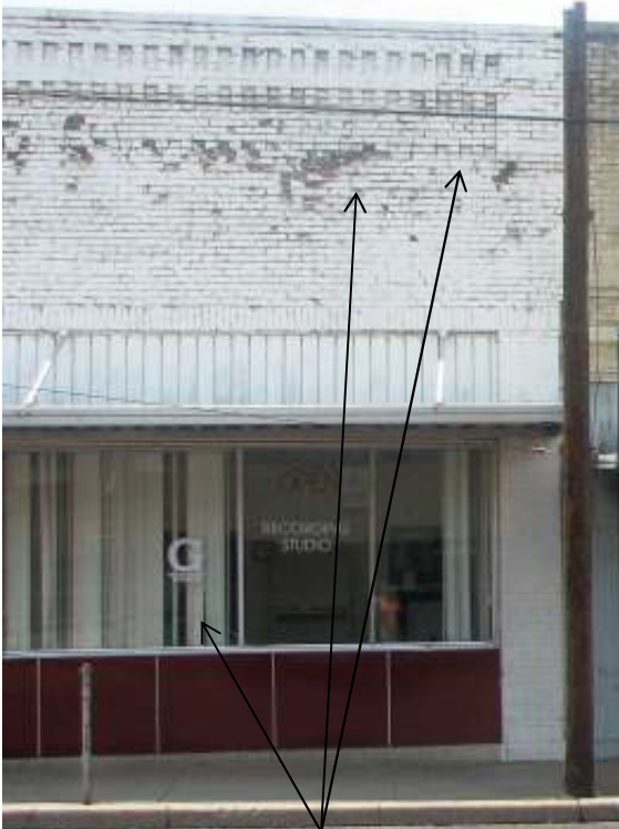
Façade (207) showing cracked window, peeling paint and mortar issues
