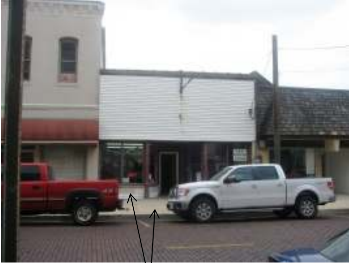
Façade (north), showing missing vinyl siding panel
