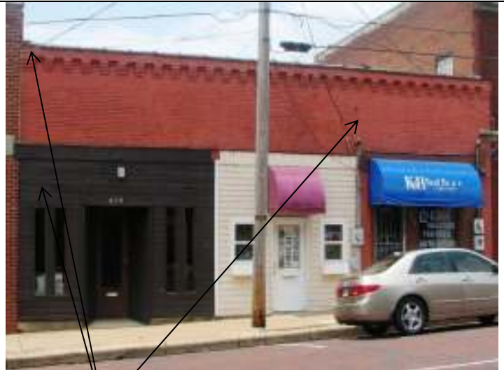
Façade, showing loose wood siding, loose (trim) coping, and areas of cracks in mortar
