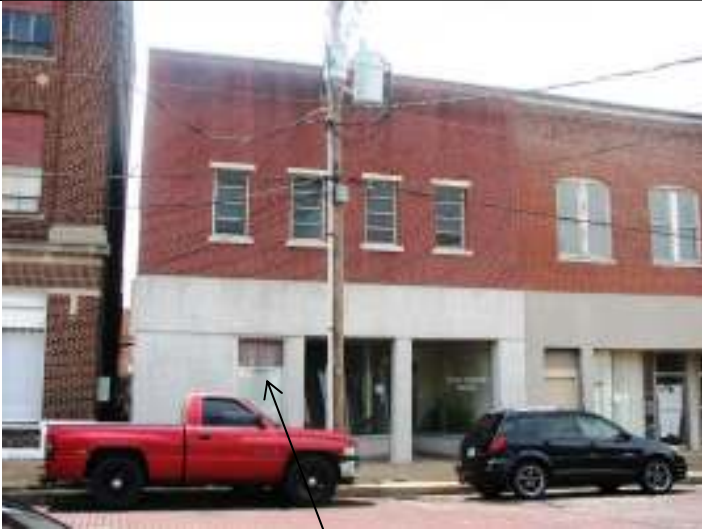
Façade (east), showing infilled window opening
