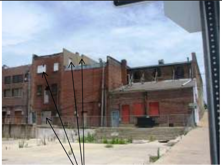
West and south elevations, showing boarded up windows and doors, and cracked stucco
