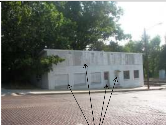
Façade and south elevation, showing boarded windows, missing glass panels in doors, and worn metal slip cover.
