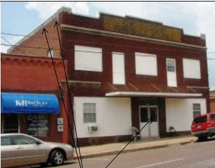
Façade and south elevation, showing improper re-pointing of the brick, missing brick, broken window in door, and enclosed window openings
