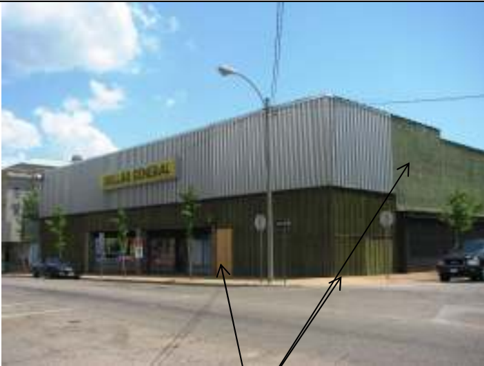
Façade (west) and south elevation, showing missing storefront window, deteriorated wood siding, and peeling paint
