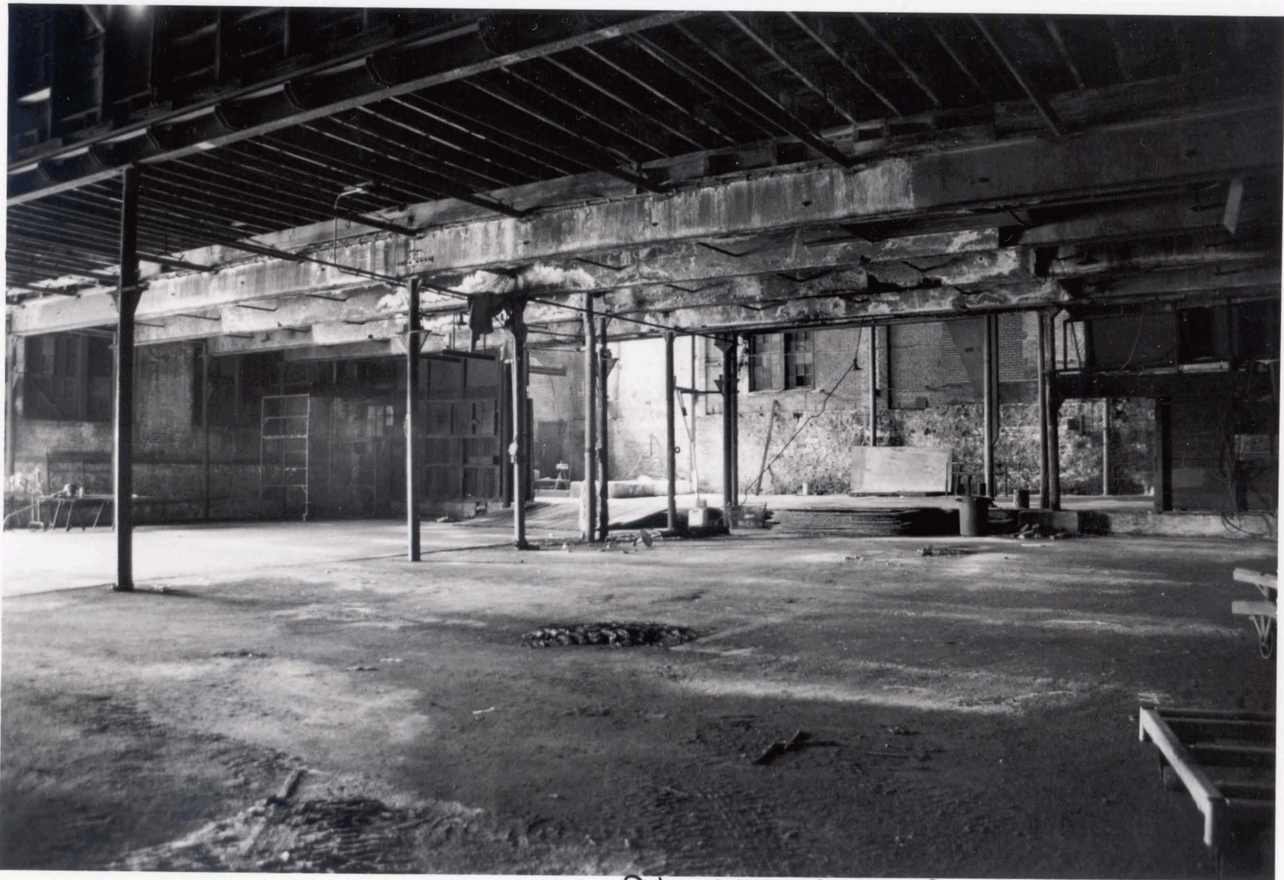
Polar Wave Ice and Fuel Company, Plant No. 6 St. Louis (Independent City) MO. Photo # 8
