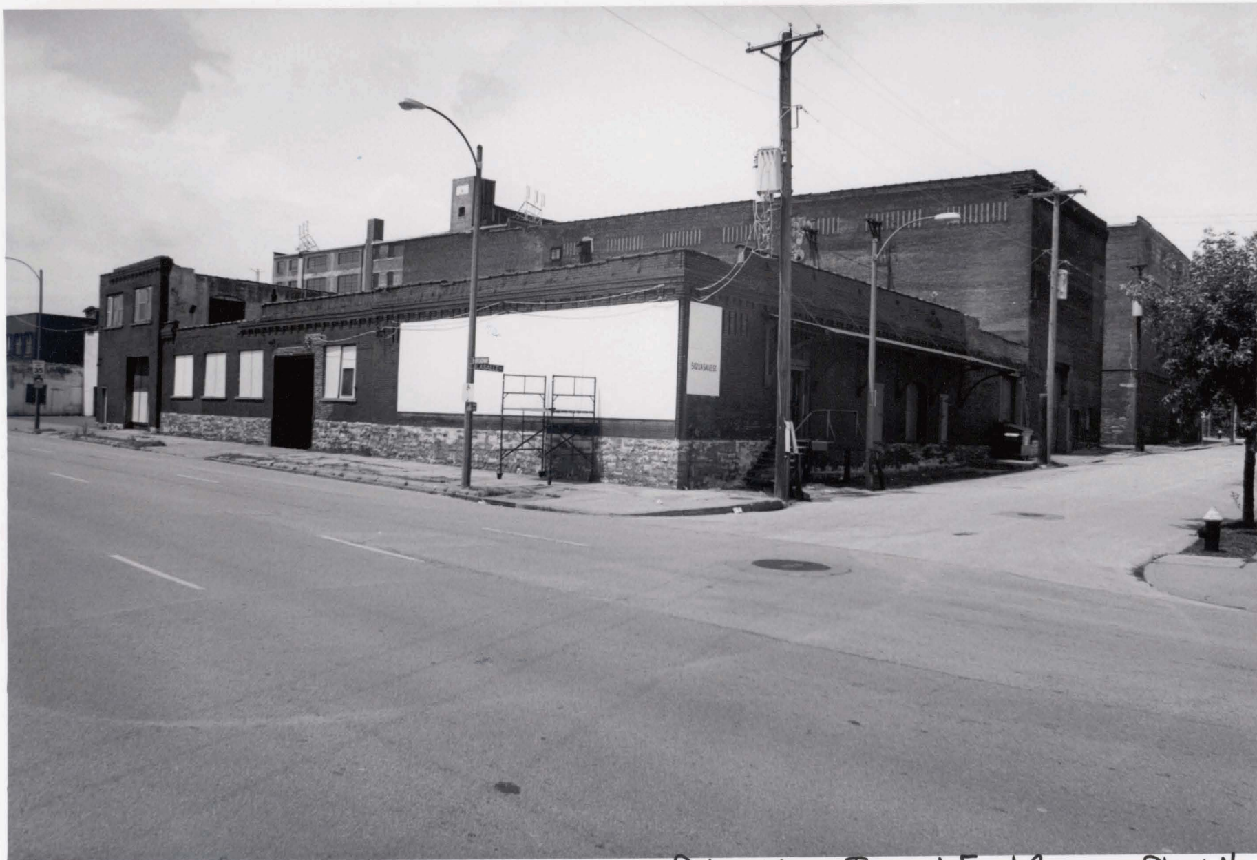
Polar Wave Ice and Fuel Company, Plant No. 6 St. Louis (Independent City) Mo. Photo # 1
