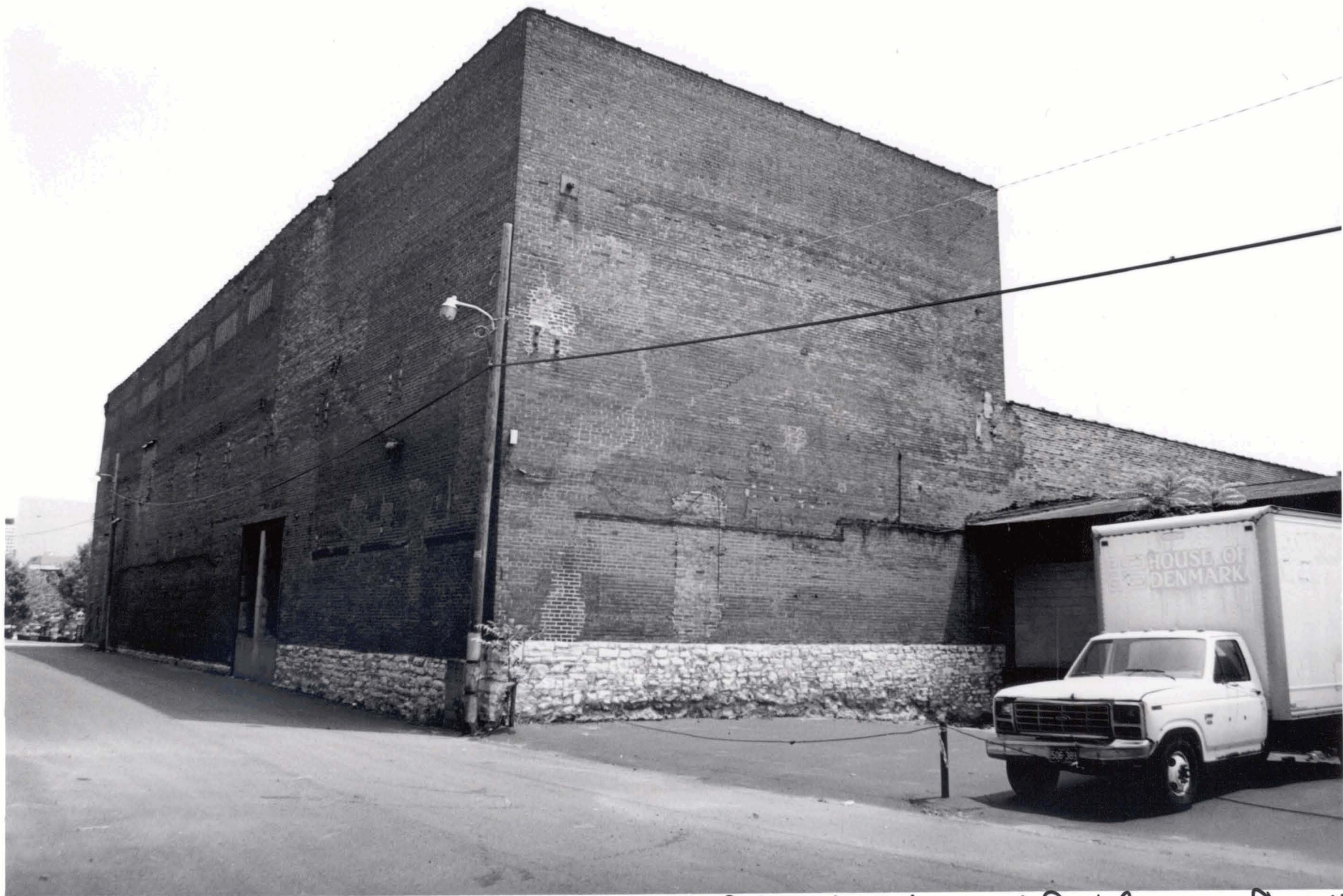
Polar Wave Ice and Fuel Company, Plant No. 6 St. Louis (Independent City) Mo. Photo # 4
