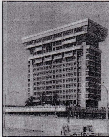
Figure 16: Equitable Building (1969) 200 South Fourth Street
