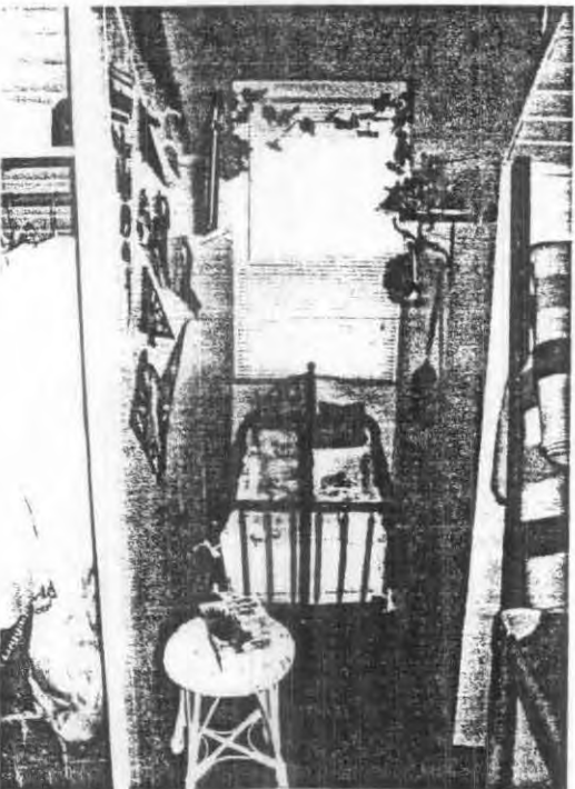
Detail of dormer in attic
