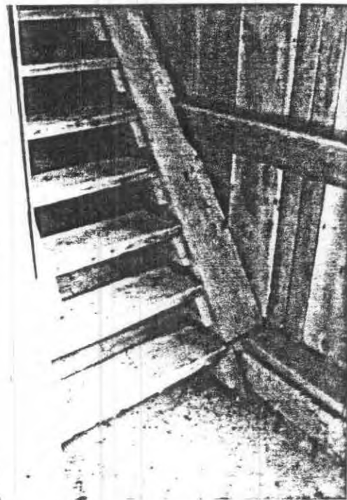
Detail of stair
