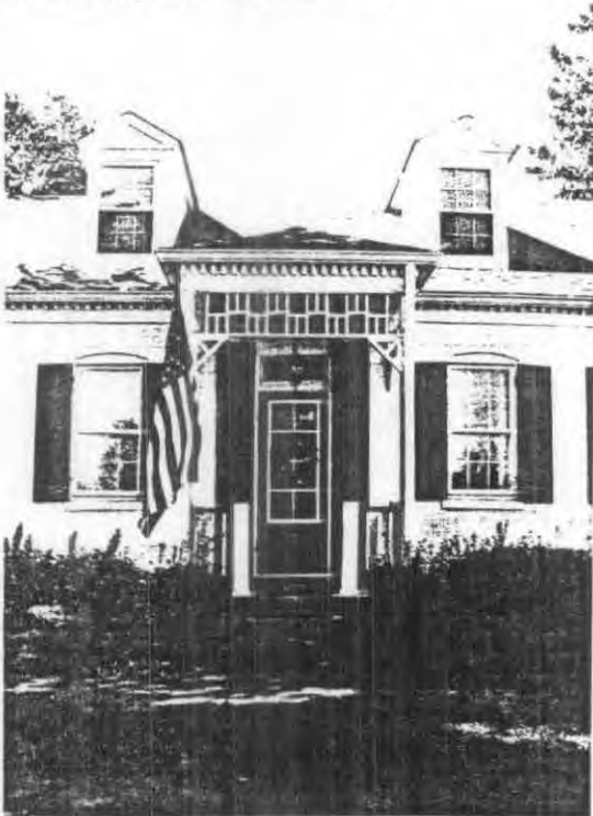
Center bays of East Elevation
