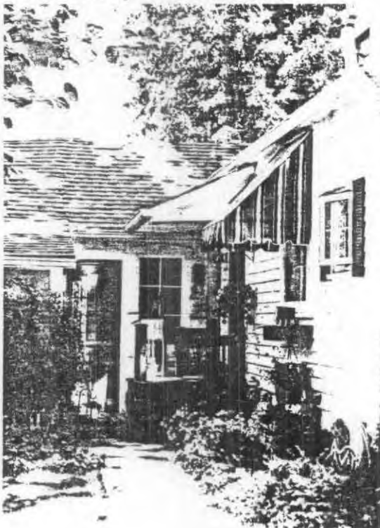
Detail of rear porch & Breezeway
