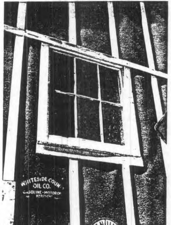
Detail of window of East Façade
