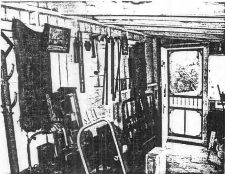
Interior View to Southwest
