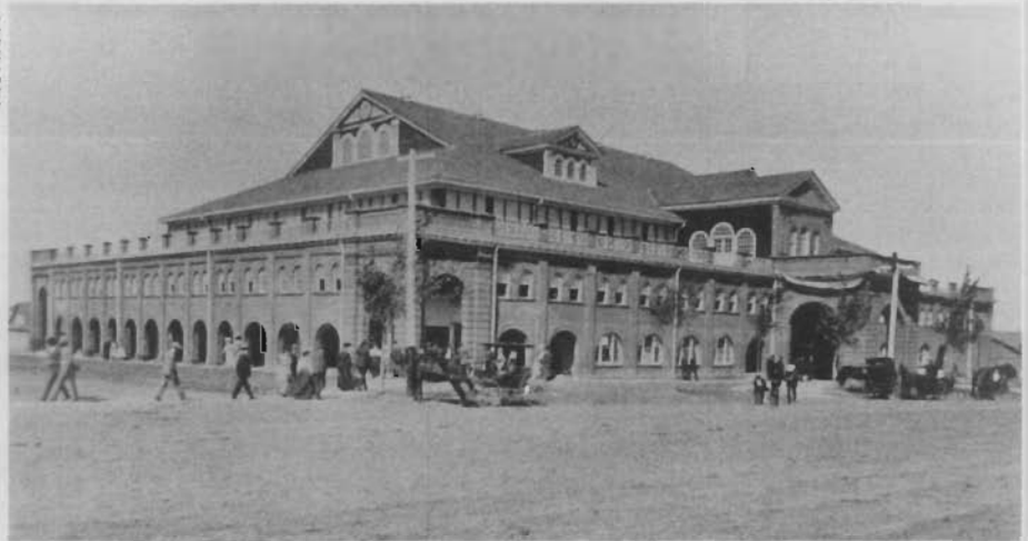
Live Stock Pavilion shortly after construction.
