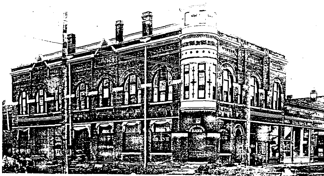
Picture of Opera Hall Block c. 1920
