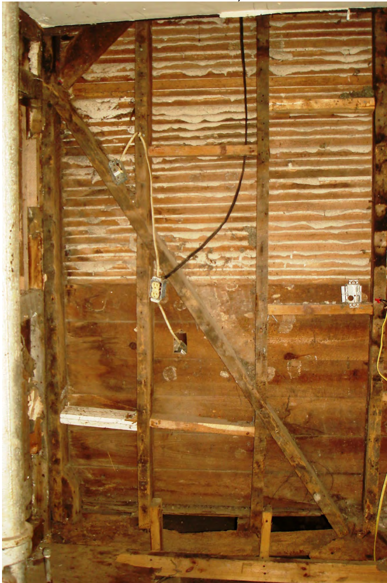
12 of 17: Room 101, interior framing of the east wall. (Photo taken in 2012, before the rear additions were removed.)
