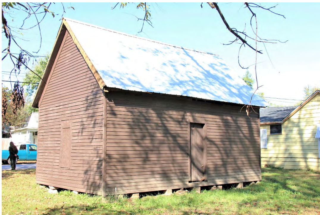
4 of 17: Southeast corner.
