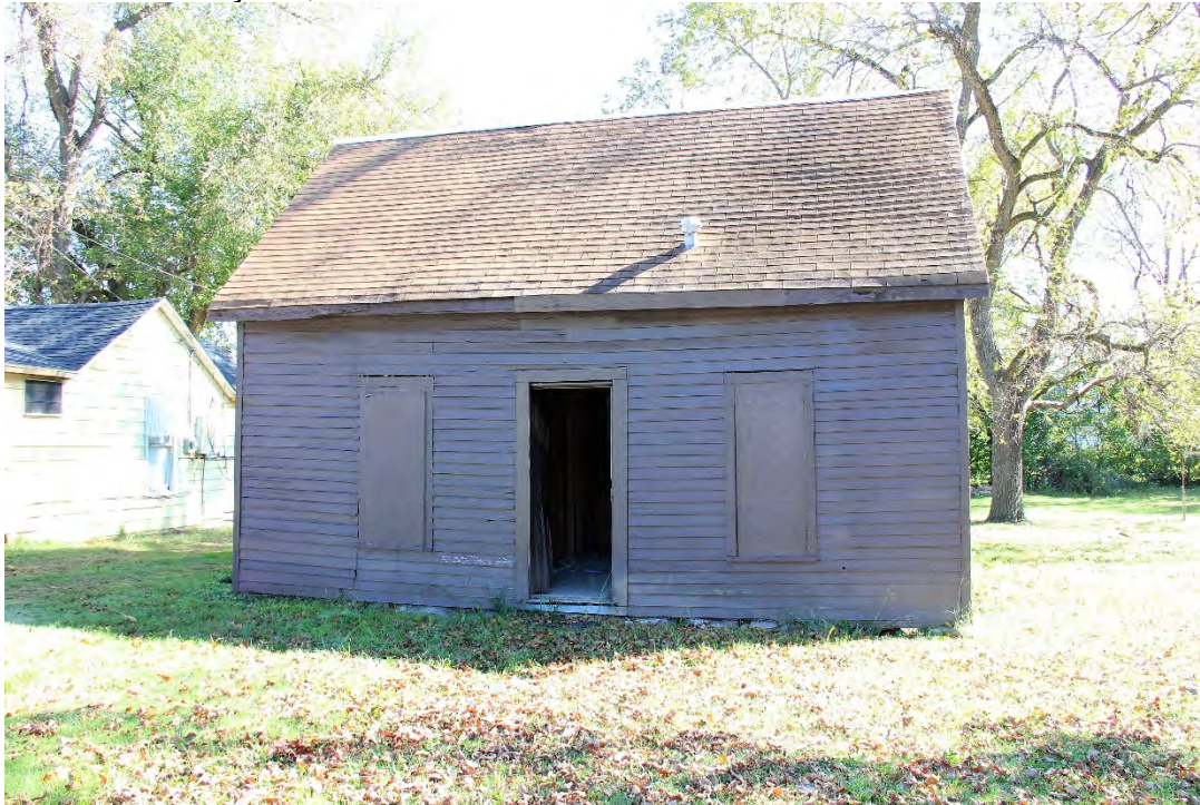
1 of 17: Façade, west wall.
