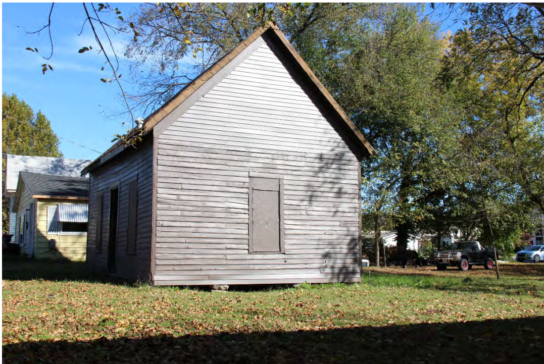
2 of 17: South side wall.
