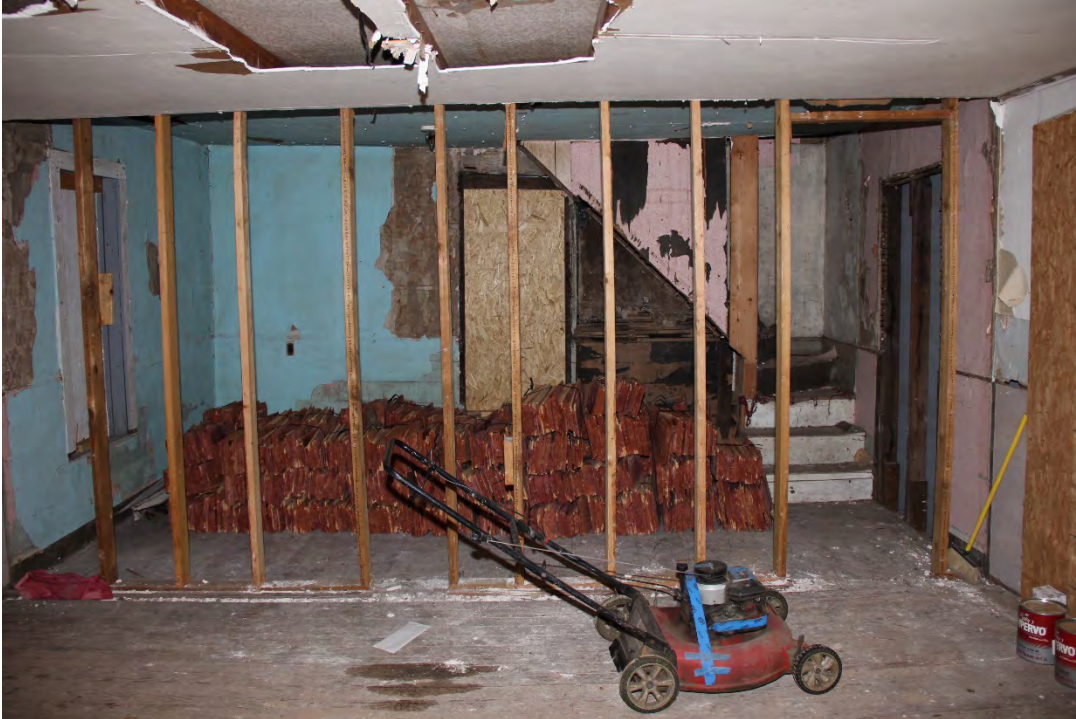
15 of 17: Room 102, looking north from Room 101.
