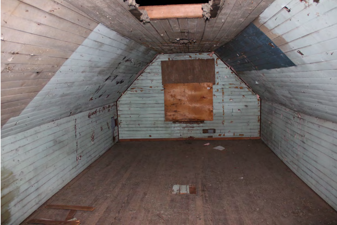
17 of 17: Room 201, looking south, (second floor).
