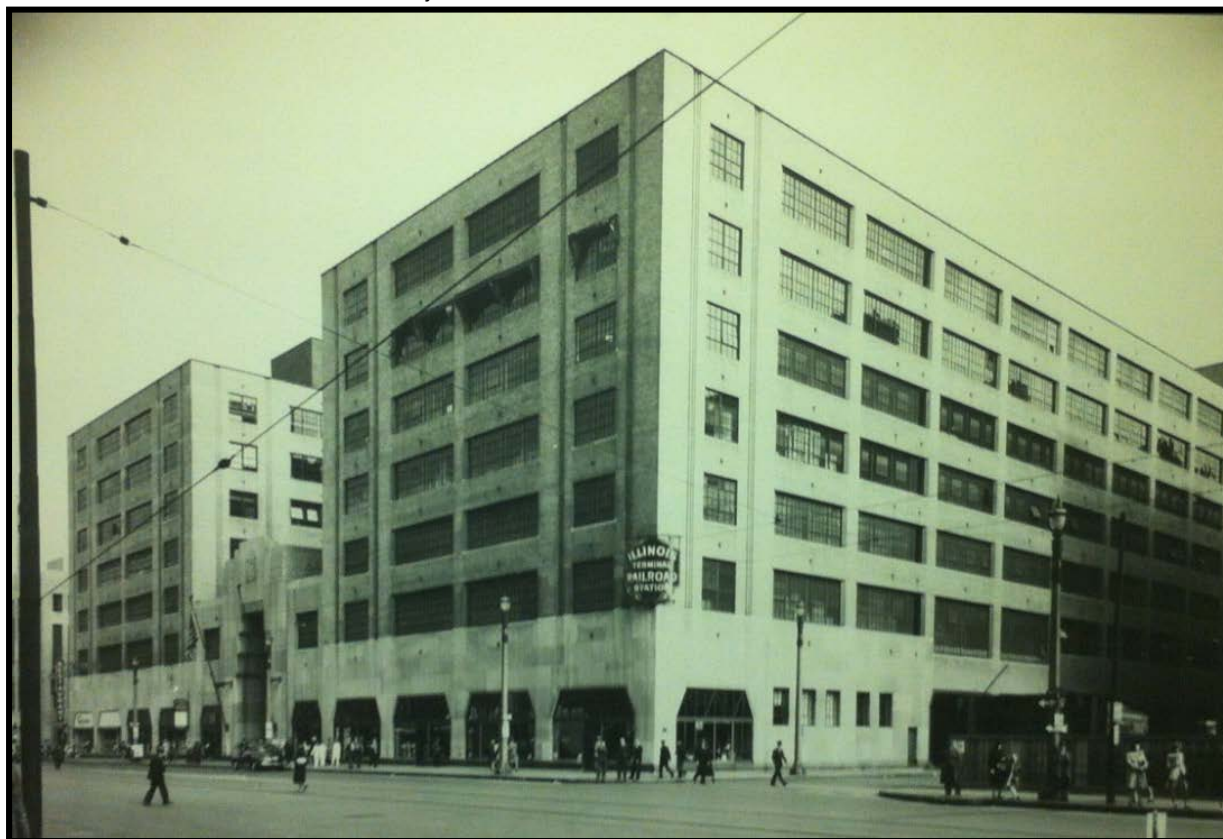
Figure 27: October 1942 photograph of the Midwest Terminal Building, view to northeast. Source: Aeronautical Chart Maintenance Project, St. Louis, Missouri. Exhibit A, 10-24-1942.
