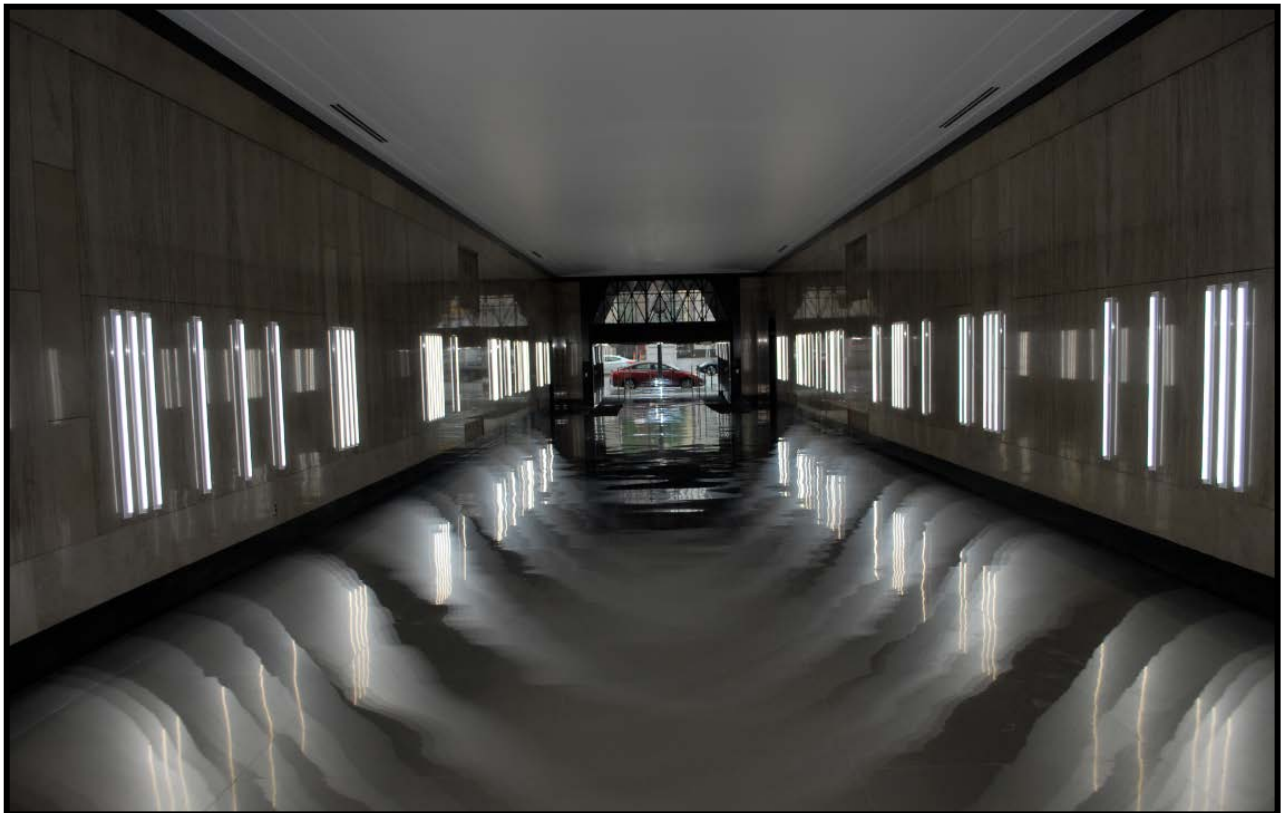
Figure 7: 1 st floor hall looking west towards North Tucker Boulevard. Original terrazzo floor is intact beneath metal floor veneer; vertical lighting is removable but provides light in an otherwise dark corridor. Source: Matt Bivens photograph, 2015.
