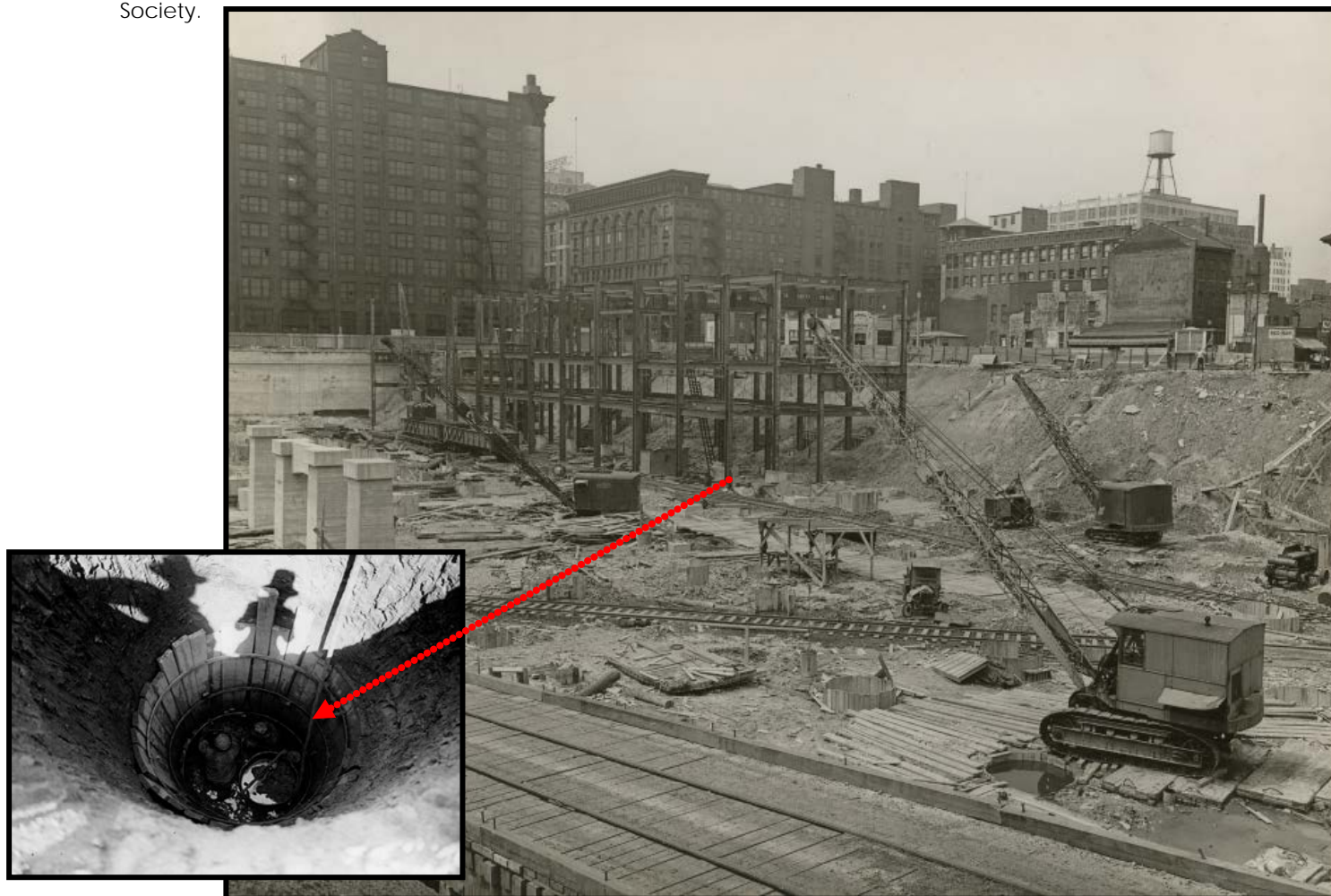
Figure 22: Photograph of building construction site facing southwest towards Washington Avenue and 12 th Street with steel framework of the terminal building raised above ground on July 4, 1931 (top). At the far left side is the Carleton Building (since demolished) and to its right is the Ferguson-McKinney Dry Goods Store and Warehouse (NR listed Washington Avenue Historic District 2-12-1987). The smaller image at the bottom left shows the men whom sunk down below surface to hand dig the piers for the structural columns. Source: TOP-Collection of Dale Jenkins, Illinois Traction Society; BOTTOM-Collection of Missouri Historical Society.
