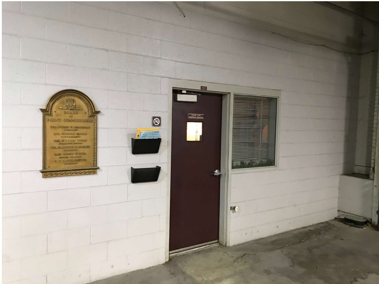
Figure 22: Current view of partition wall at east side of vehicle entrance. Source: Preparer photograph, March 2020.
