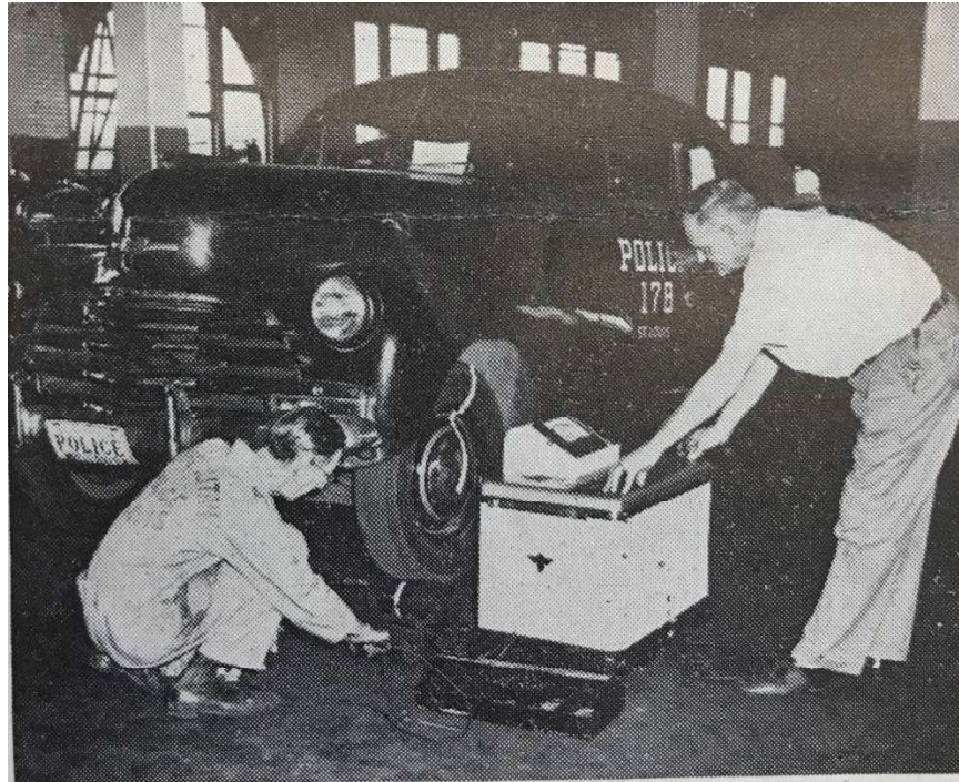
Max Hartzke, mechanic, and Anthony Nies, shop foreman, of the Police Garage use the electronic wheel balancer.
