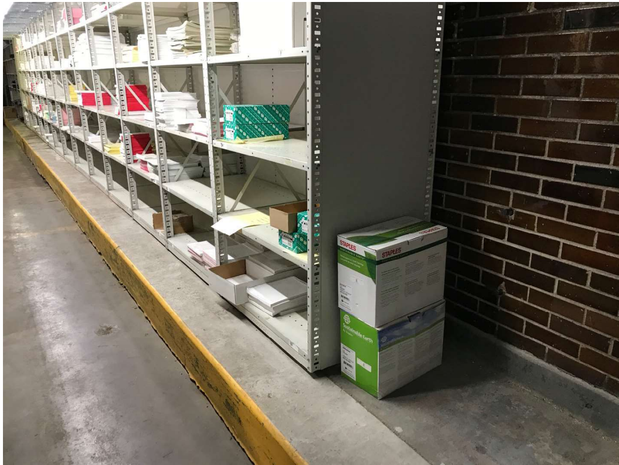
Figure 30: Current view of intact curb on east side of first floor. Source: Preparer photograph, March 2020.
