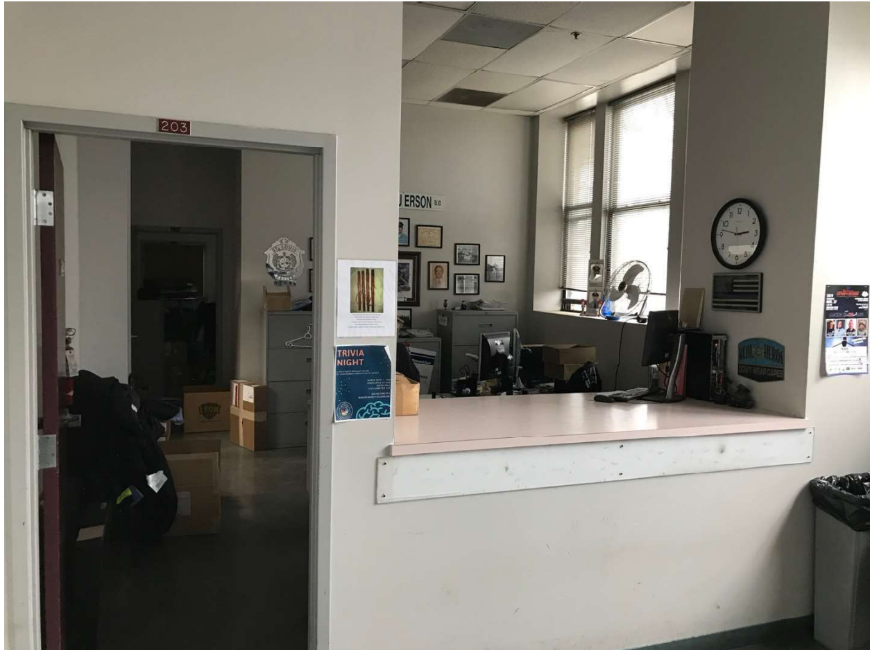
Figure 32: Current view of second floor office area. Source: Preparer photograph, March 2020.
