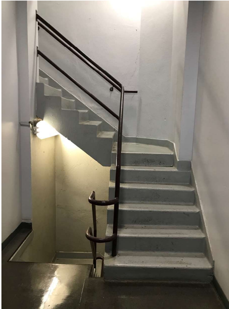
Figure 23: Current view of staircase at lobby. Source: Preparer photograph, March 2020.
