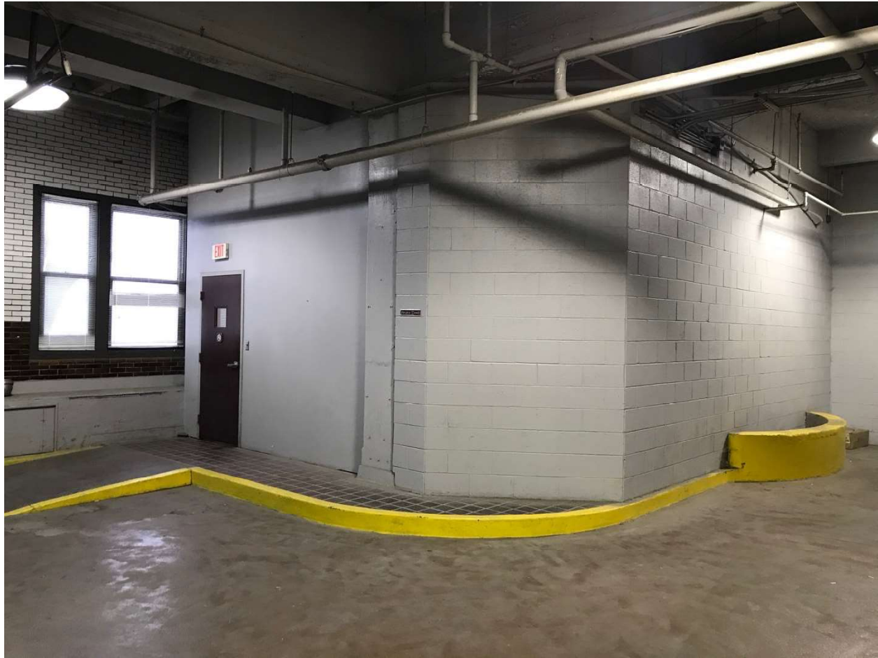
Figure 29: Current view looking toward lobby opening from the vehicle lane. Source: Preparer photograph, March 2020.
