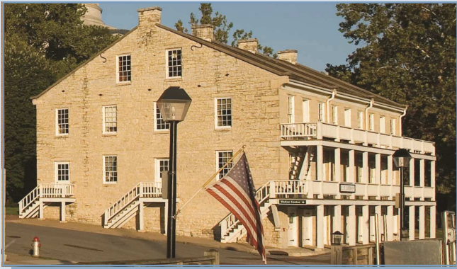
The Lohman Building is open until Aug. 31, 2014. Come help us celebrate this building's 175th birthday!
