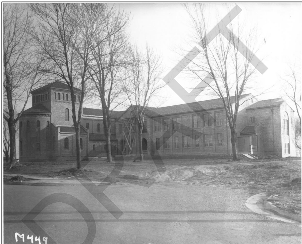
Figure 10. High School and Seminary under construction, 1930. Source: Missouri Valley Special Collections, Kansas City Public Library, Kansas City, Missouri.
