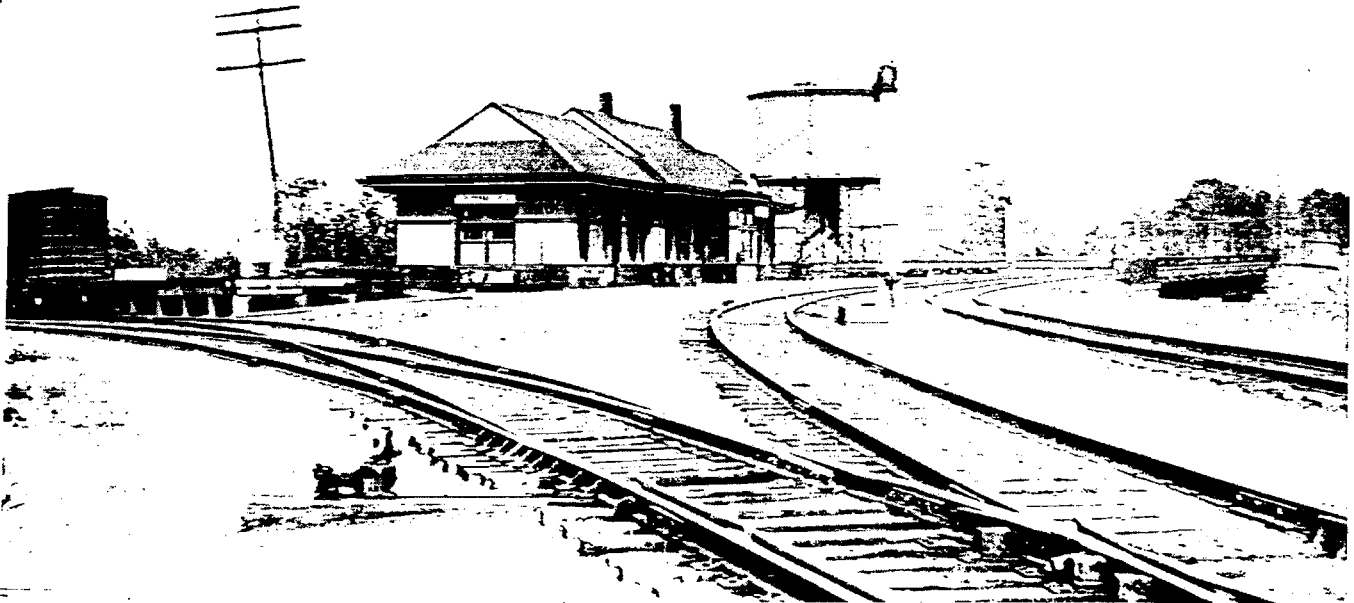
GOLF MUEHLE + CHIC DEPOT ALTON RAILROAD - SHOWING WATER TANK + CRANES MAY 1947
