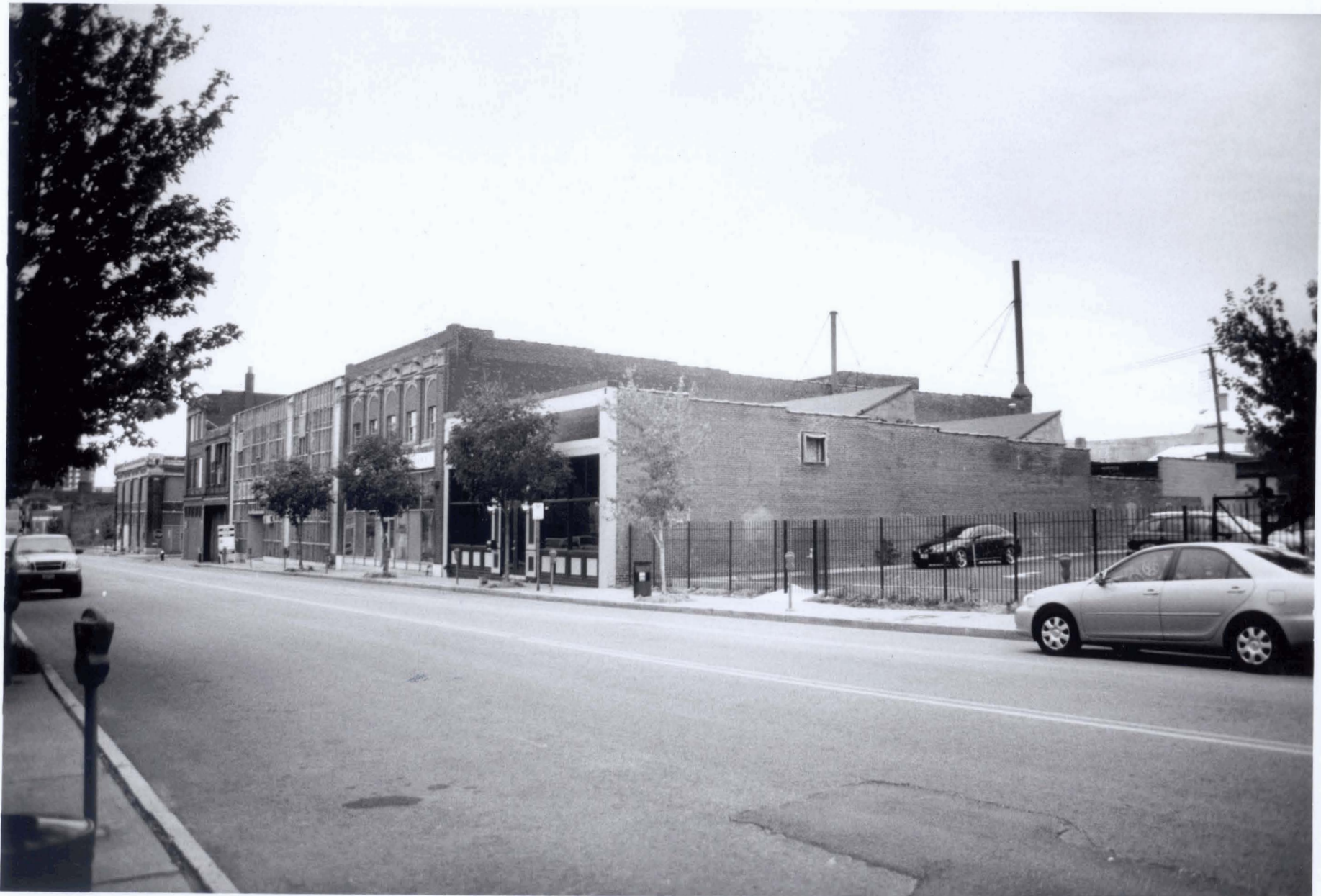
Locust Street Automotive District (Boondary Increase) St. Louis (Independent City), MO Photo No. 1
