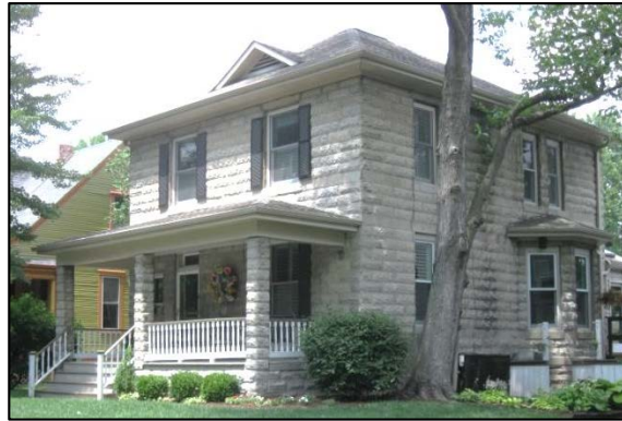
1504 Watson Street, circa 1907. This Pyramidal form house/American Four Square is unusual as it is built of rock-faced concrete blocks and rather than a dormer it has a vented gablet on the front slope of the roof.
