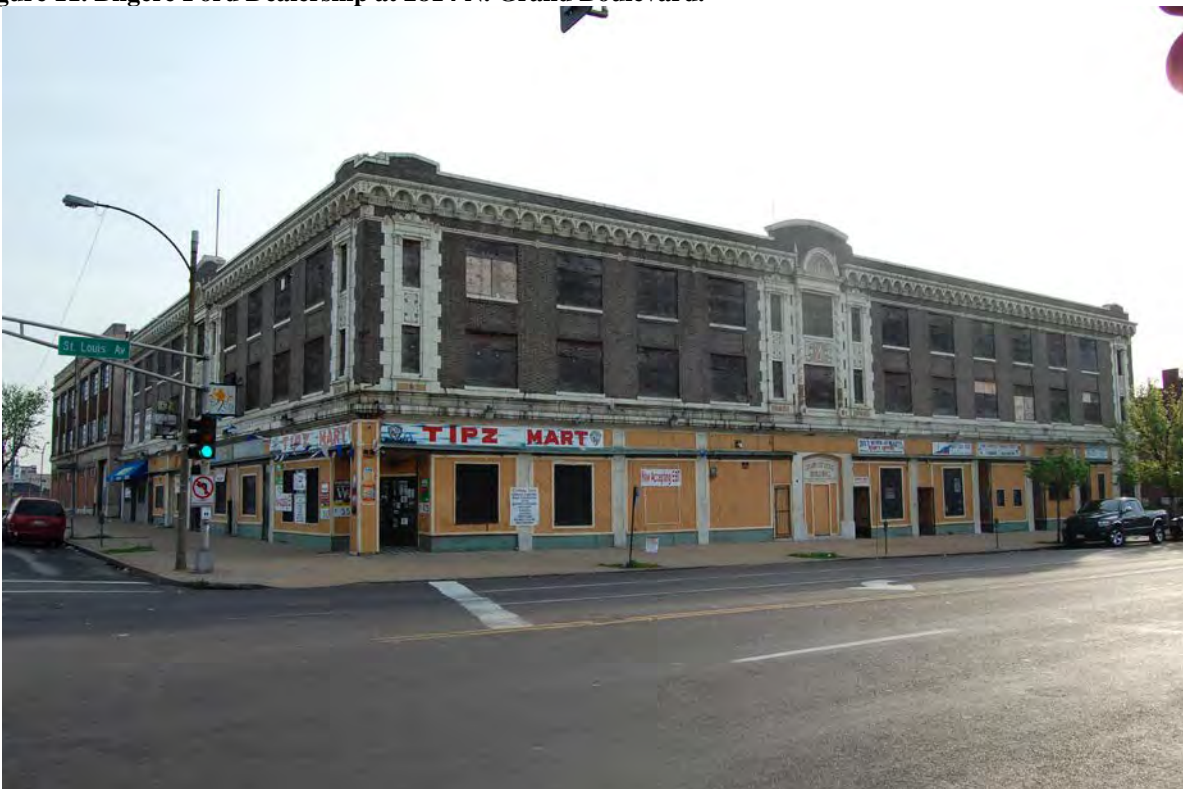
Figure 12. Grand-St. Louis Building at the northeast intersection of St. Louis Avenue and N. Grand Boulevard
