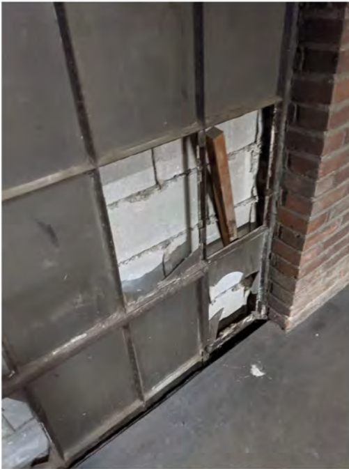
Figure 15. Detail photos of concrete infill installation from interior. Top: Note the air cavity between steel window frames and masonry infill. Bottom: Note that modern exterior louvers are placed within the concrete blocks, and steel window frames remain intact in a parallel plane. Photos by Homegrown Studio, 2021-2022.
