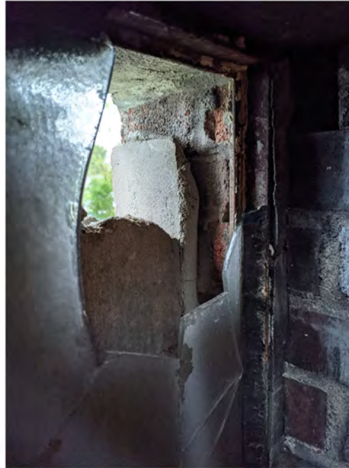
Figure 15. Detail photos of concrete infill installation from interior. Top: Note the air cavity between steel window frames and masonry infill. Bottom: Note that modern exterior louvers are placed within the concrete blocks, and steel window frames remain intact in a parallel plane. Photos by Homegrown Studio, 2021-2022.
