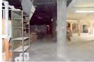
THIRD LEVEL LOOKING EAST
