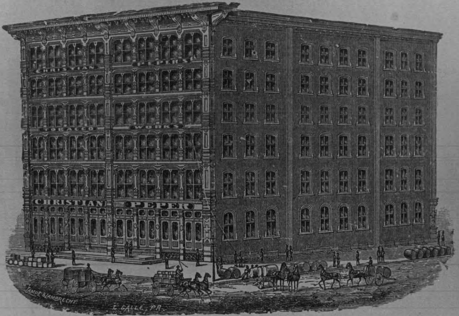
THE PEPER BUILDING.
