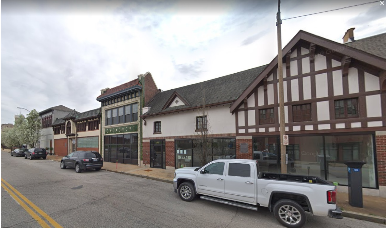
Figure 21. The 2900 block of Locust Street Automotive District exhibits the district's Tudor and Spanish Revival influences (Source: Google Maps, 2020).
