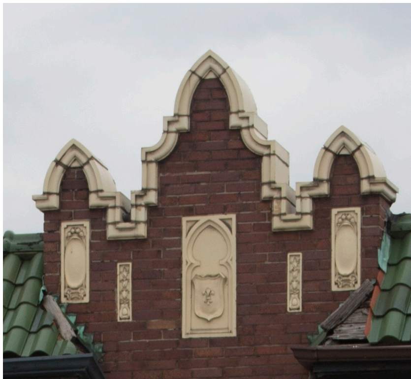
Figure 16. 3801-03 S. Kingshighway has Moorish-inspired motifs such as ogee-shaped arched parapets and decorative terra cotta panels (Photo: Keenoy, April 2019).
