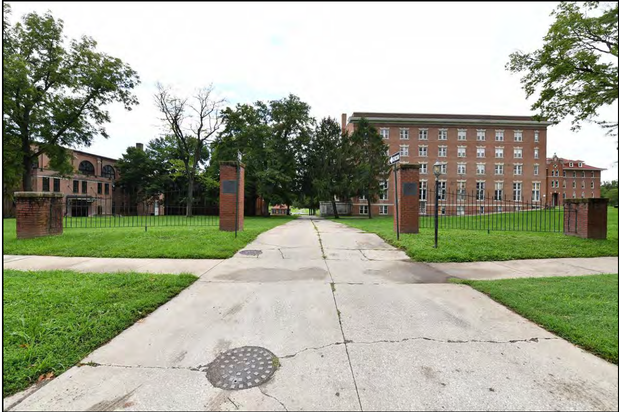
Figure 27: Southeast Gate ( Resource 34 ), looking west from 3 rd Street (Brad Finch, f-Stop Photography, 2023).
