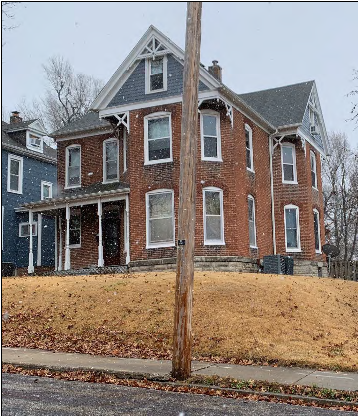
Figure 31: Kusgen-Melkersman Residence (Mason Martel, 2023).
