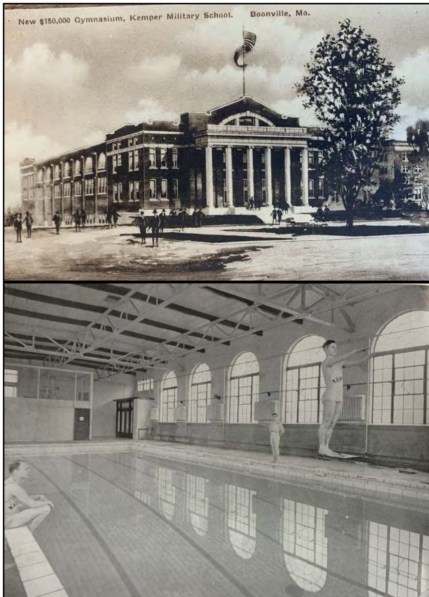
Figure 11: Top: Undated (likely ca. 1925) postcard of the Johnston Field House; Bottom: 1939 photo of the interior of the Pool Annex (“New $150,000 Gymnasium, Kemper Military School, folder 7, Kemper Military School (Boonville, MO.) Collection (C4174) ); Kemper Military School, View Book (Boonville, Missouri: Kemper Military School, 1939), no page. Kemper Military School Museum Archives).
